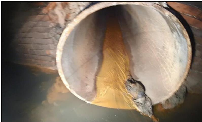
**Figure 2-8. View of 30-inch Dry Weather Flow Pipe Protruding into Regulator RE-081**
