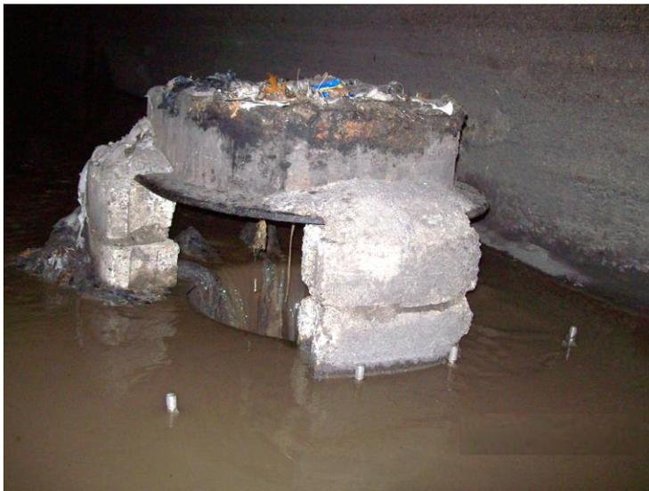
Figure 6-1. SOM001A, RE01A Hydraulic Restriction
