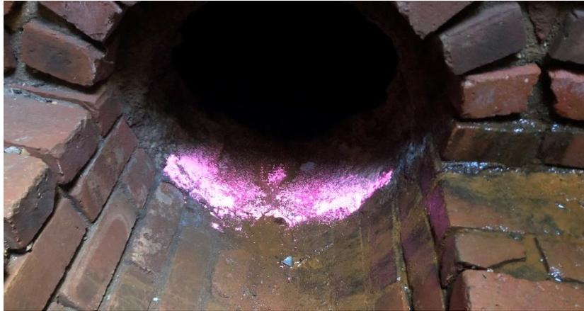
**Figure 4-3. Chalking Applied to the Overflow Pipe at RE070/8-8**
