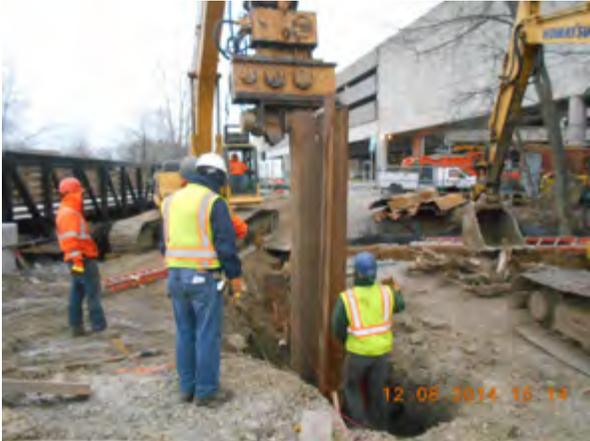
**Installation of Steel Sheet Piling for Excavation Support
