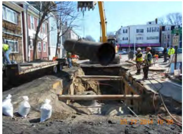
**Installation of 48-inch Drain on E. Third Street
