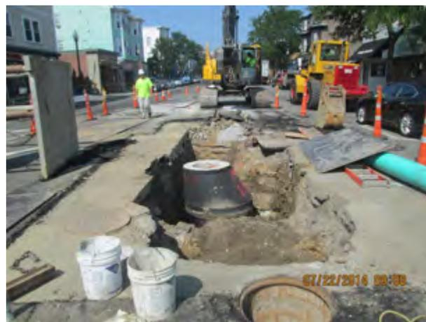
**12-inch Storm Drain Installation on East Broadway
