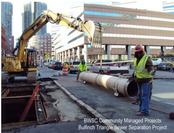
Installation of storm drain on Causeway Street
