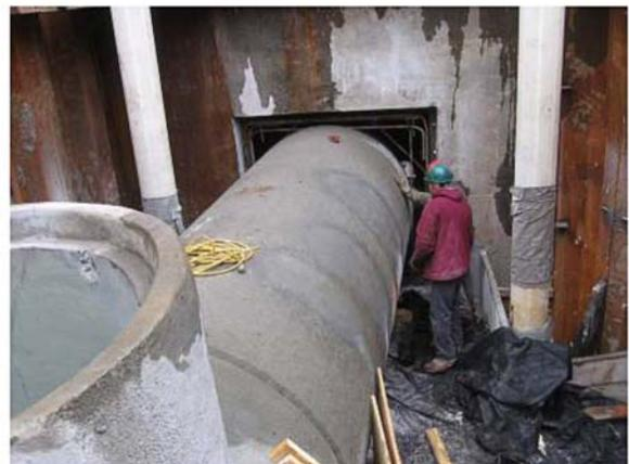
New 60-inch PCCP pipe interconnection between the North & South Charles Relief Sewer overflow chambers in the Cottage Farm yard.
