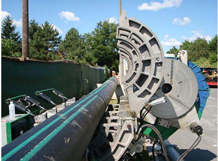
East Boston Branch Sewer Interceptor Relief Contract 3: Pipe Bursting 16" diameter pipe fusion HDPE on Marginal Street, East Boston
