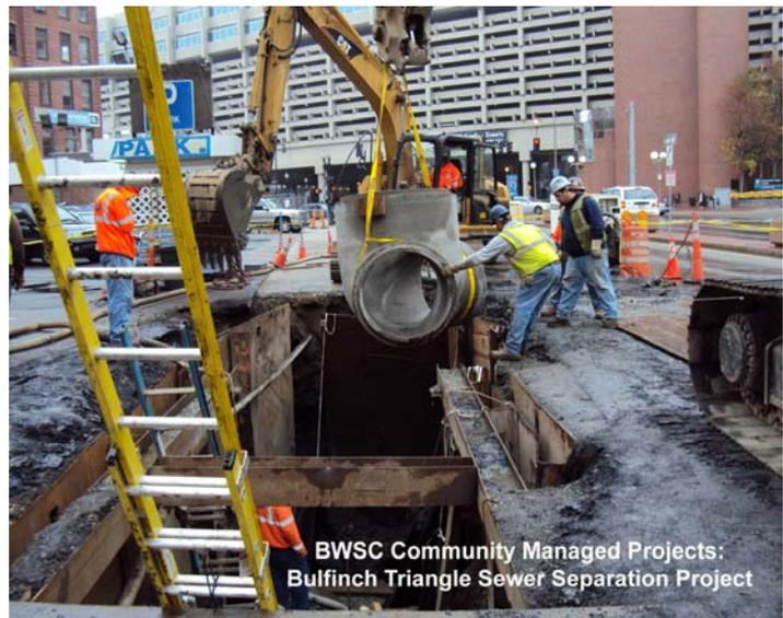
**Installation of storm drain on Merrimac Street**
