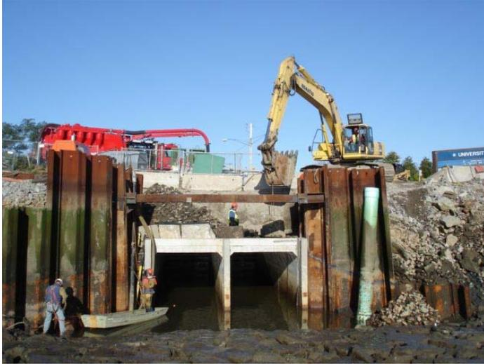
In March 2006, MWRA completed construction of the Pleasure Bay storm drain improvements, ending wet weather discharges to Pleasure Bay Beach and physically removing a dozen storm drain outfalls along the beach. The project relocated the Pleasure Bay stormwater discharges to the less sensitive Reserved Channel, which is primarily a shipping channel.
