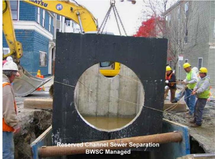
**Installation of special manhole at East Second and O Streets**
