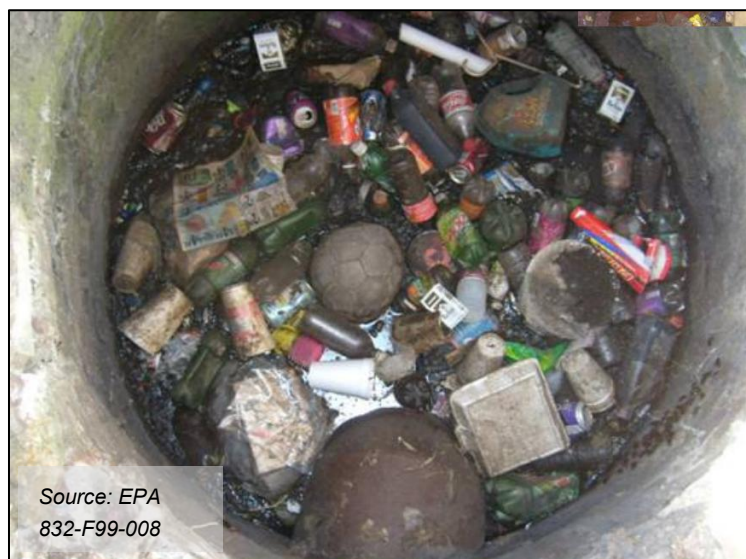
Figure 2-2 Catch Basin Hood with Floatable Material
