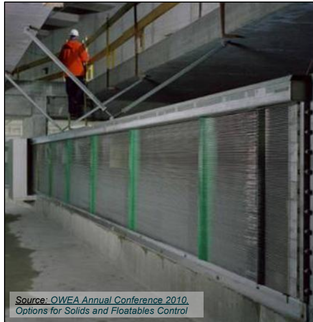
Figure 2-4. Example of Mechanically cleaned Horizontal Bar Screen
