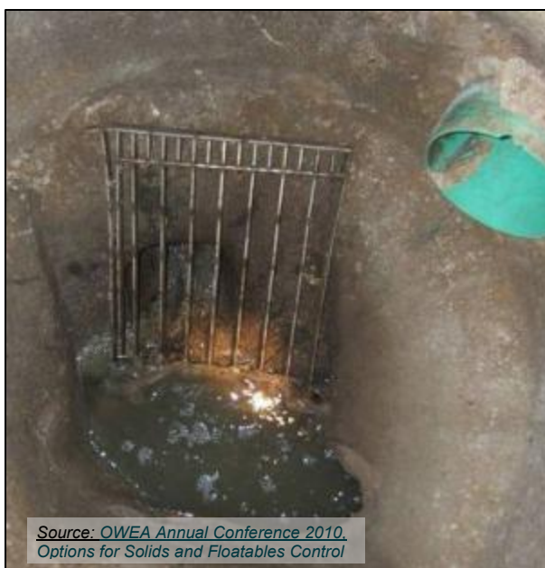
Figure 2-3 Manually cleaned Trash Rack in a Combined Sewer System
