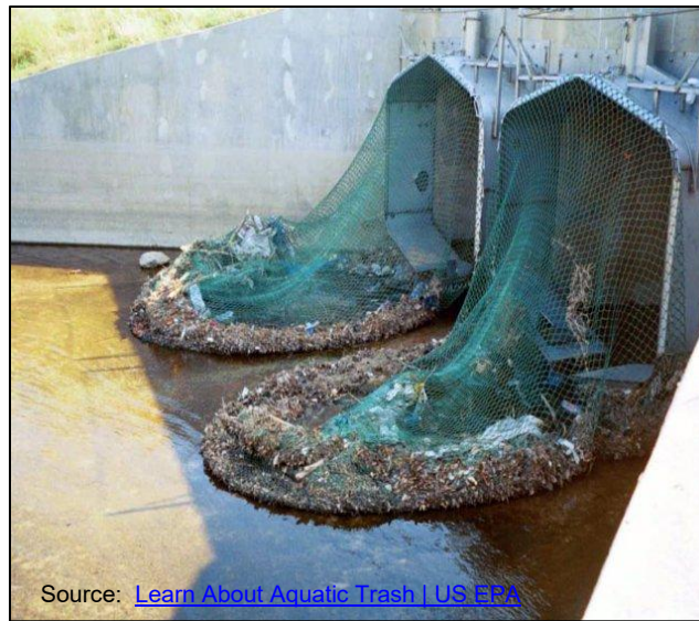
Figure 2-7 End-of-Pipe Netting at an Outfall
