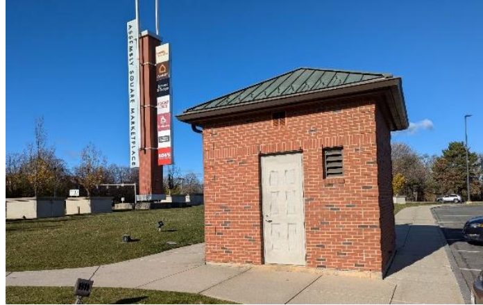
Figure 6-2. MWRA Somerville Marginal CSO Treatment Facility Remote Sampling Building
