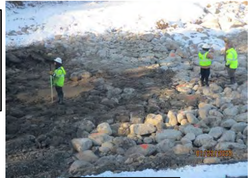
Checking riverbed grades
