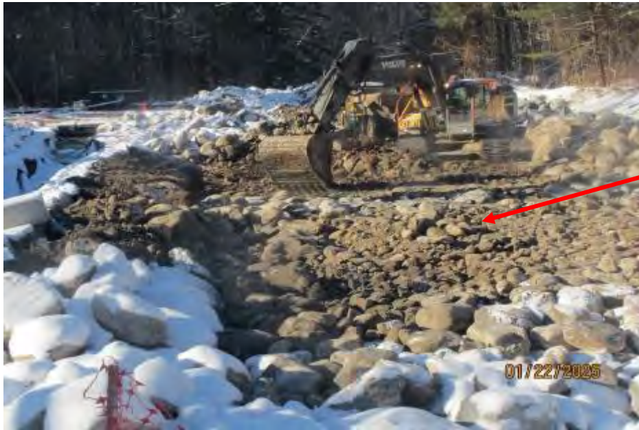
Placement of rock for riverbed riffle
