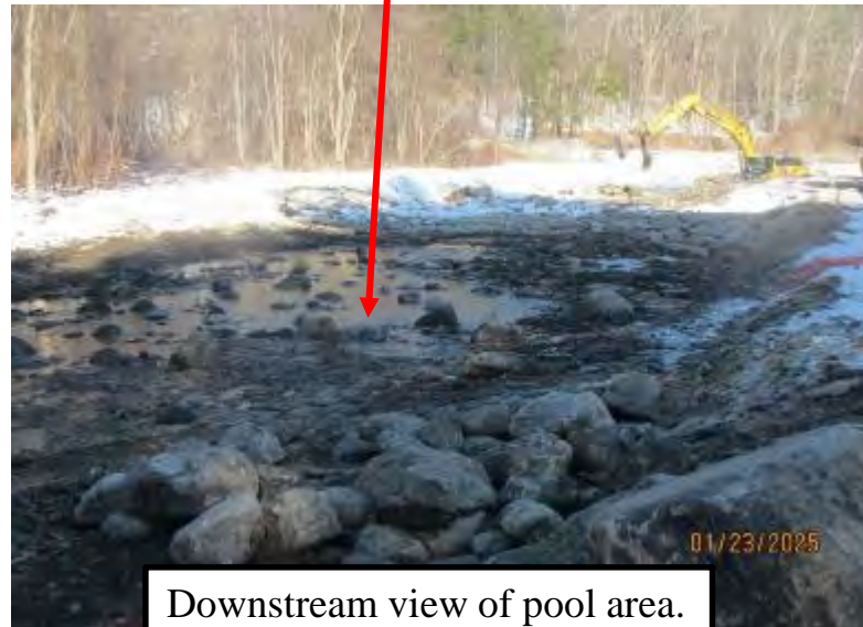
Placement of rock for riverbed riffle
