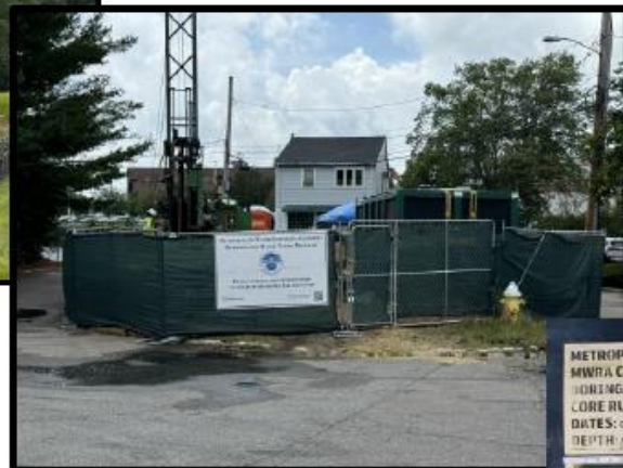
Deep Boring Site Set-up
