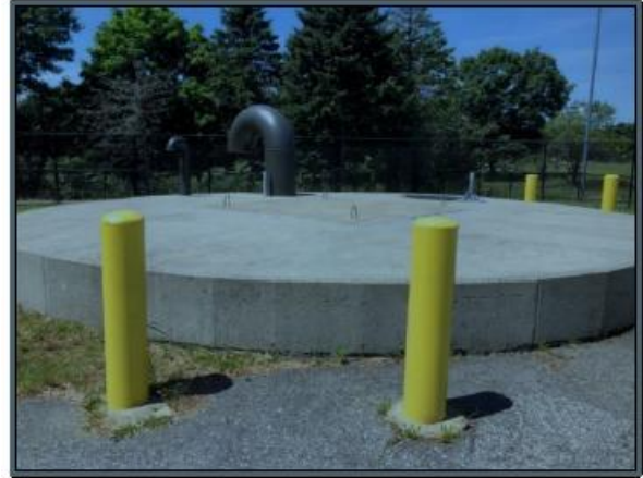
MWWST Shaft 5/5A, Weston
