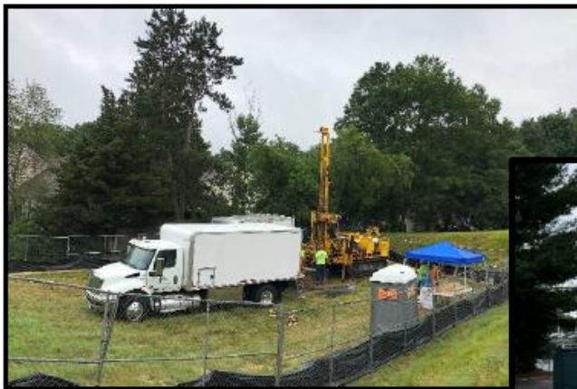
Deep Boring Site Set-up
