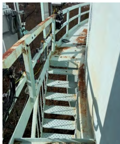
Figure 3: Corroded Stairs and Guardrail
