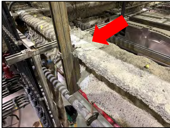
New fireproofing patches at new conduit support
