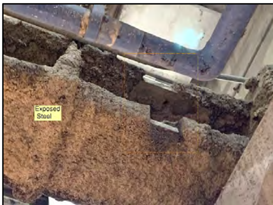
Existing fireproofing missing and exposing structural steel
