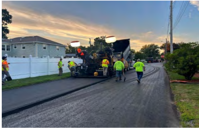
Typical reconstruction on a narrow residential road
