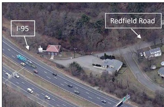
Figure 1: Hayes Pump Station Location
