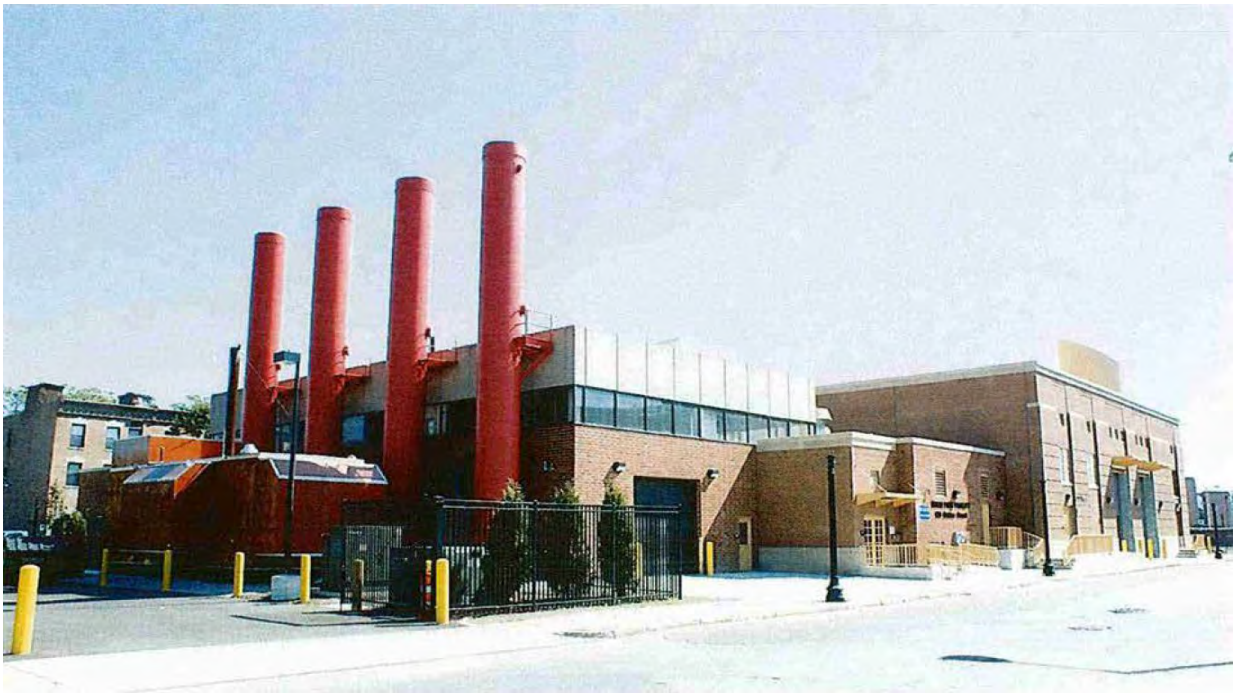
Figure 2 - Exterior View of the Facility from Malden Street
