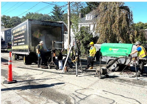
Cured-In-Place-Pipe Liner for Eight-inch Sewer on Common Street
