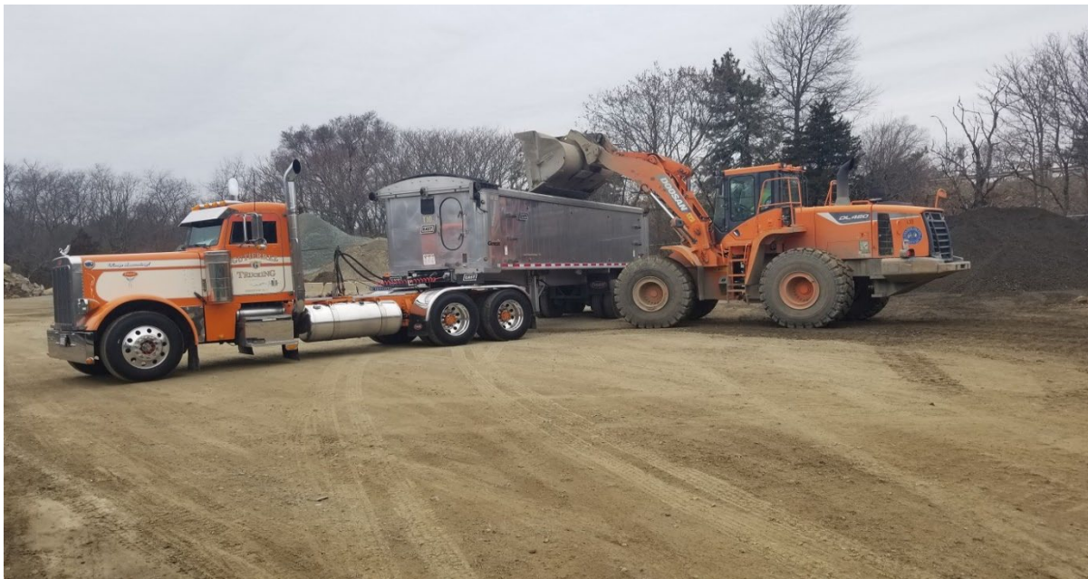
Loading soil for transport to disposal facility
