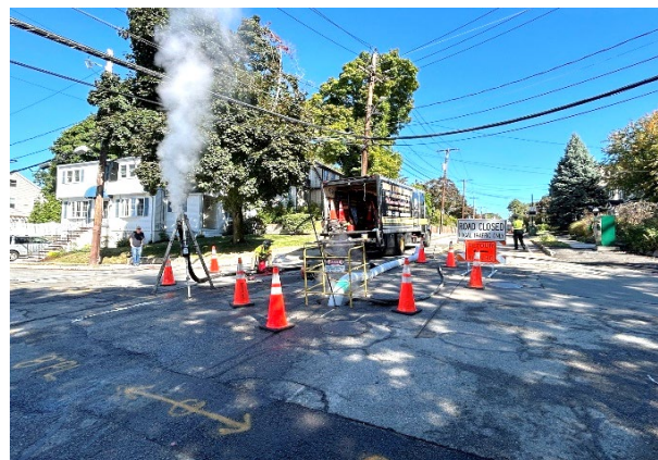
Cured-In-Place-Pipe Liner for Eight-inch Sewer on Common Street
