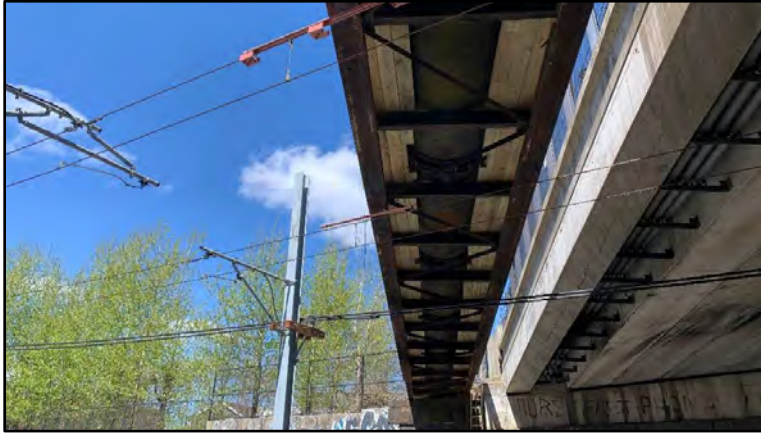
Overhead Catenary Lines under the Walnut Street Pipe Bridge
