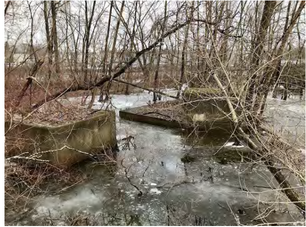
Siphon chambers subject to flooding
