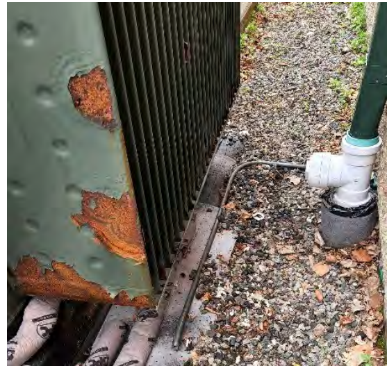
Corroded Cooling Fins on Transformer
