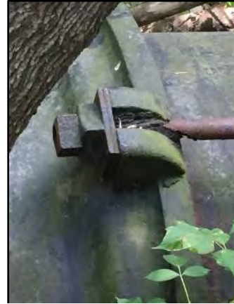
Corroded Thrust Restraint Rod
