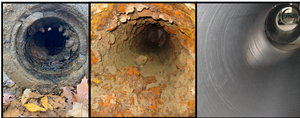
Unlined Cast Iron
