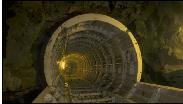
Two Pass Tunnel - Cast in Place Concrete Liner
