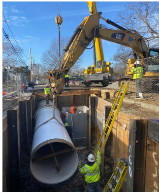
WASM 3 – pipe replacement
