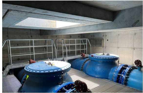
WASM 3 42-inch diameter PRVs
