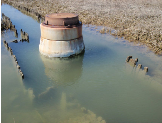
Sewer Manhole in Marsh: Raised and Sealed
