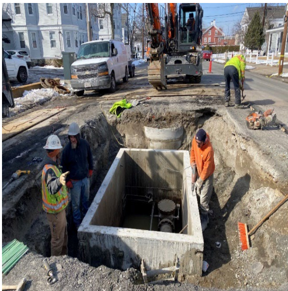
Cutting Concrete Walls at Meter 171
