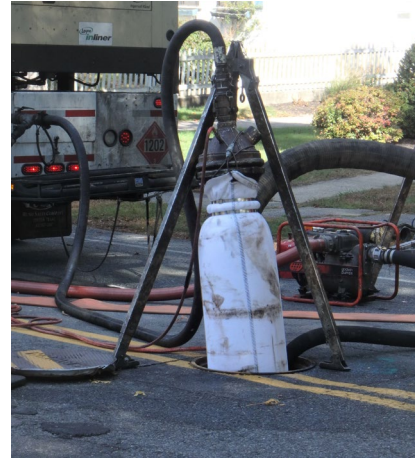
CIPP Liner Installation
