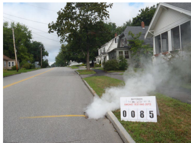
Inflow Source Identified by Smoke Testing
