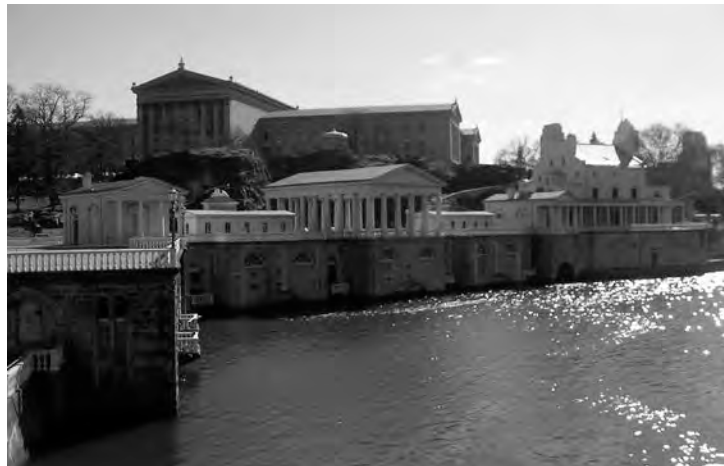
Fairmount Waterworks in Philadelphia Hydraulic pumps in the building to the right supplied water to open reservoirs on the hill where the Philadelphia Museum of Art now sits
