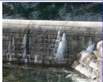
Leakage through Quabbin Spillway face
