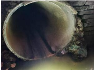
Figure 2-10. View of 30-inch Dry Weather Flow Pipe with Removed Protrusion at Regulator RE-081
