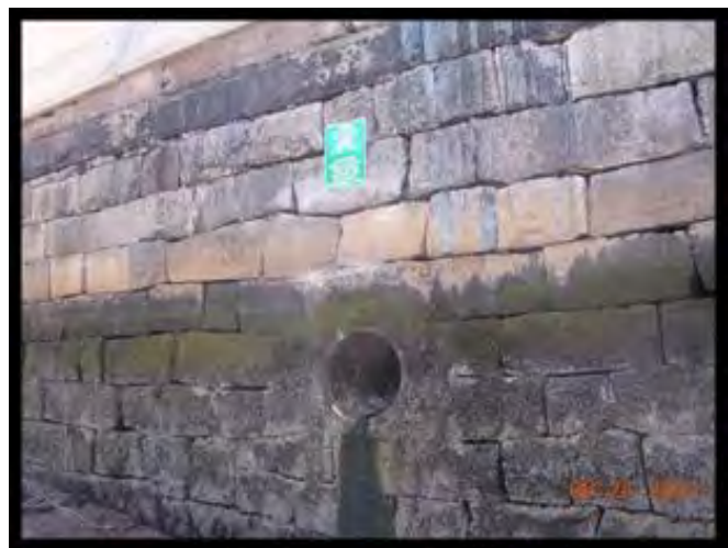
Outfall pipe below high tide water elevation of Mystic River/Chelsea Creek Confluence is now a stormwater outlet.
