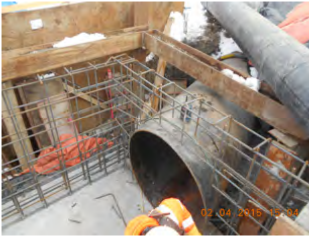
48-Inch Replacement Siphon at Outfall MWR003
