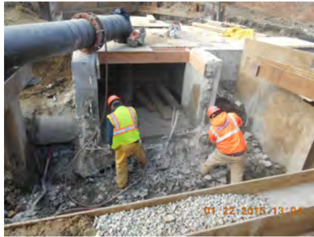
Modifications to CSO Regulator Structure RE031 at Outfall MWR003
