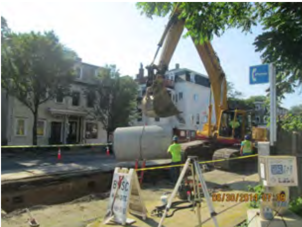
48-inch Storm Drain Installation on L Street Reserved Channel Sewer Separation Contract 4
