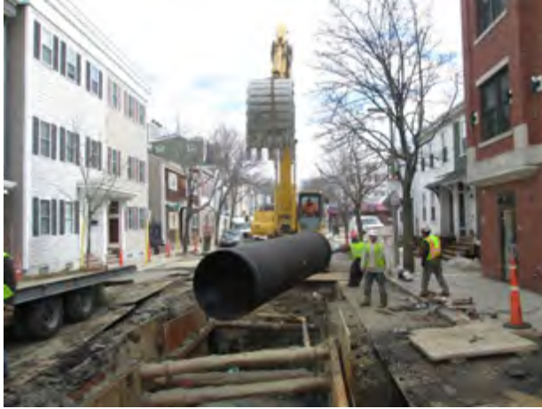
48-inch Storm Drain Installation on E. Third Street Reserved Channel Sewer Separation Contract 3B
