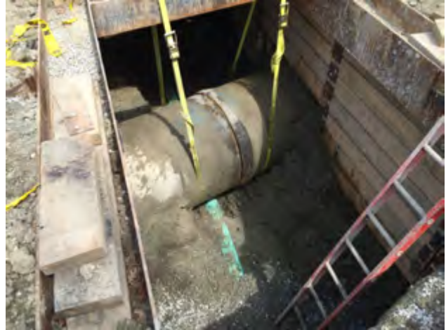
Blakeslee Street Drain Installation Under Water Main CAM004 Sewer Separation Contract 8B
