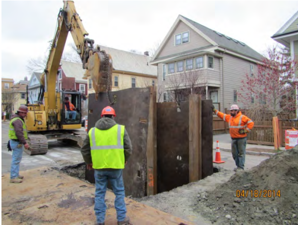
Sheeting for Drain MH on Concord Avenue Cambridge Sewer Separation Contract 9
