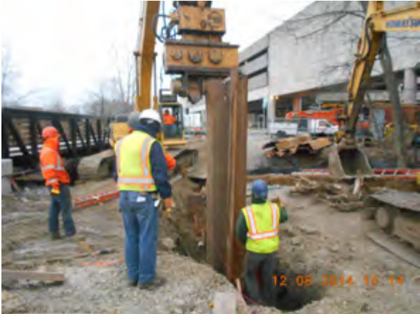
Installation of Steel Sheet Piling for Excavation Support 48-inch Rindge Ave. Siphon at Outfall MWR003
