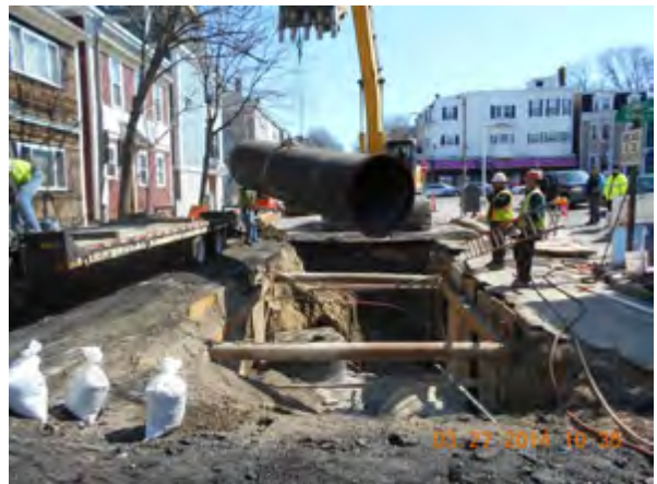
Installation of 48-inch Drain on E. Third Street Reserved Channel Sewer Separation Contract 3B
