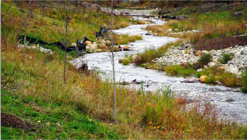
Holmes Dam Removal, Town Brook, Plymouth
