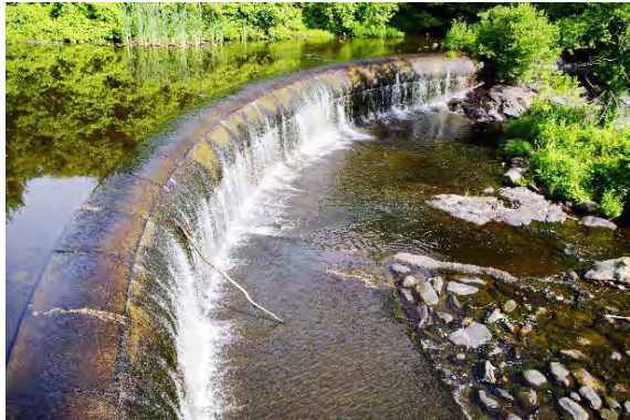
Quinapoxet River Dam
