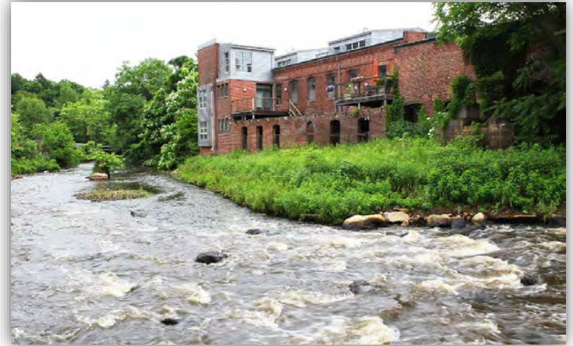
Marland Dam, Shawsheen River, Andover
