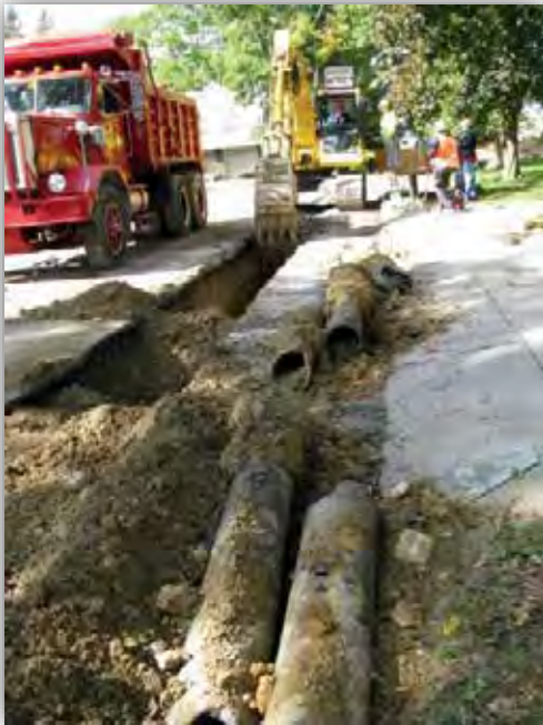
Water Main Replacement Construction
