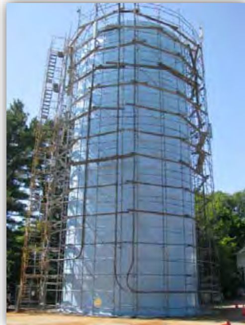
Water Storage Tank Rehabilitation
