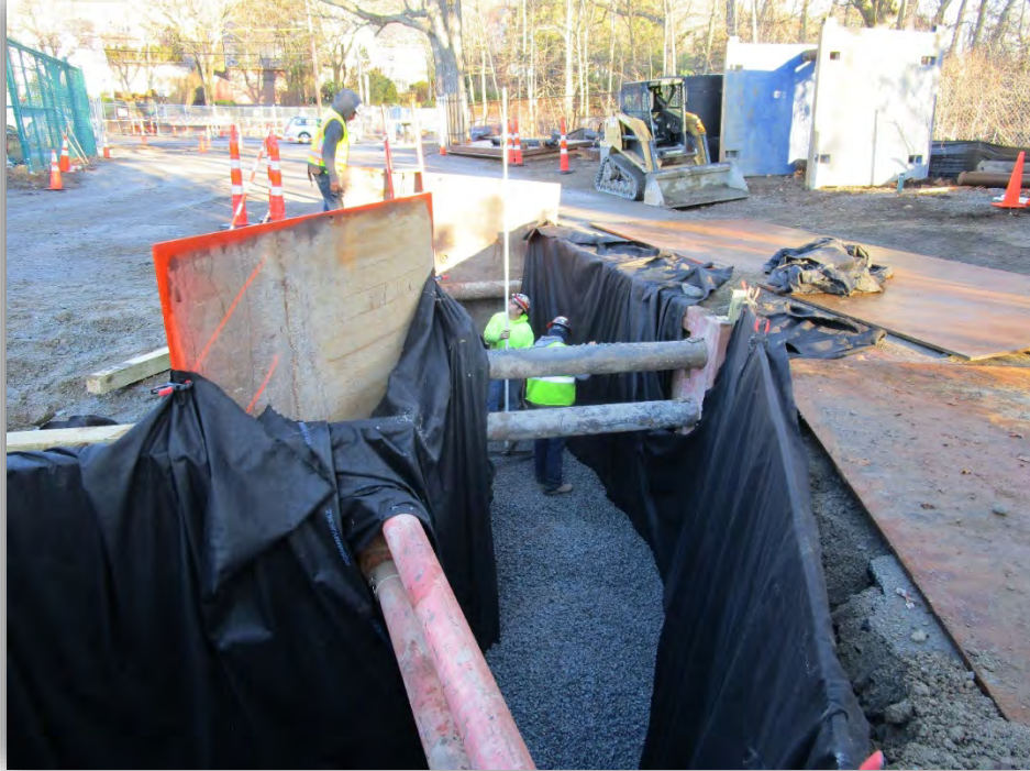
Preparing Pipe Bedding Near Valve Vault D
