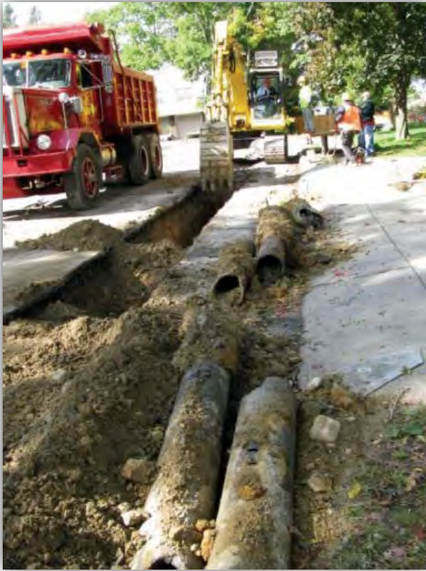
Water Main Replacement Construction
