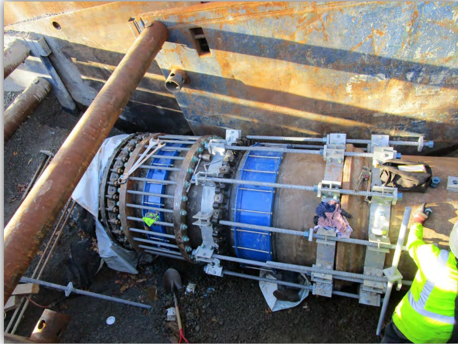
Installing Wasm1 Spool, Couplings, and Restraints
