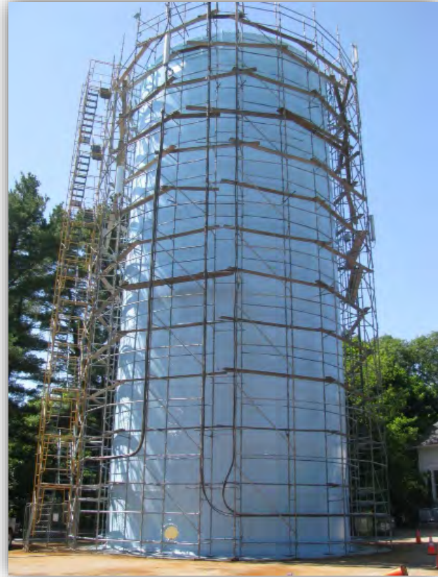
Water Storage Tank Rehabilitation
