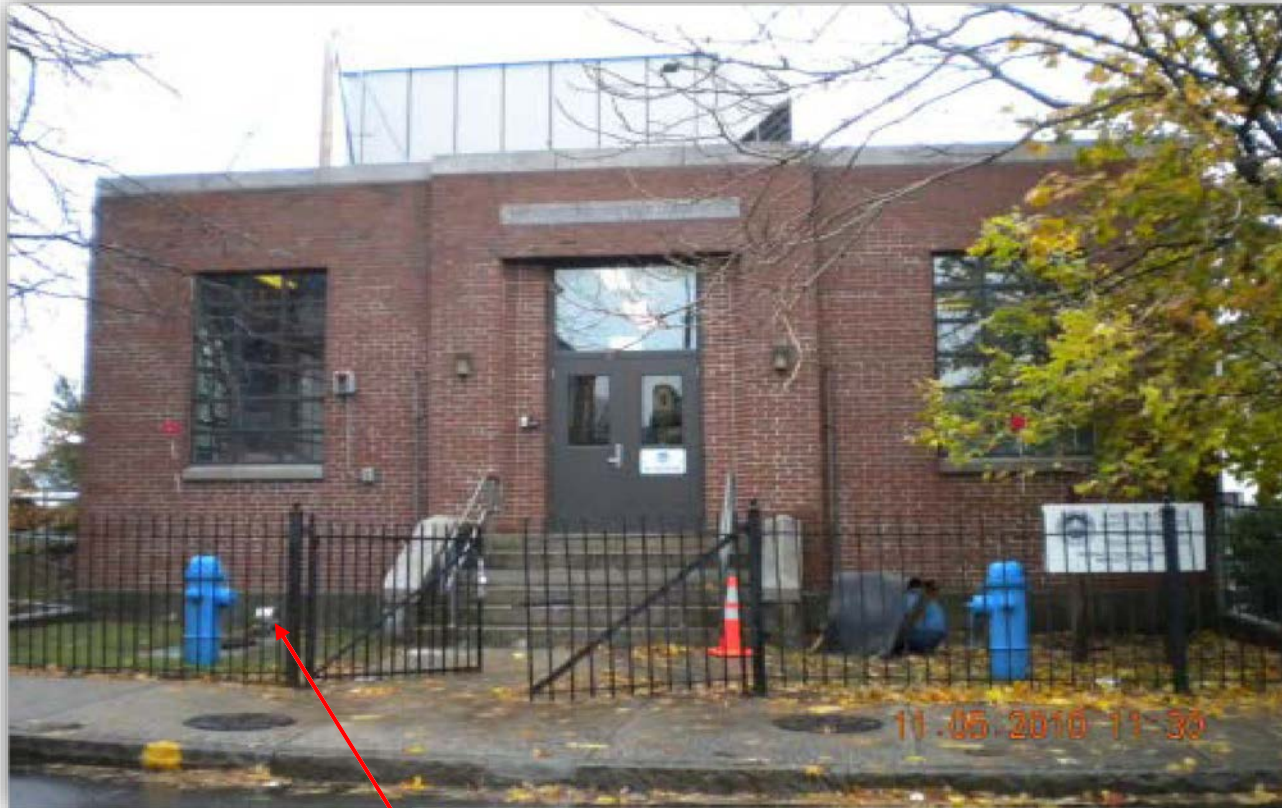
1500 GALLON STEEL TANK, 29 YEARS OLD
