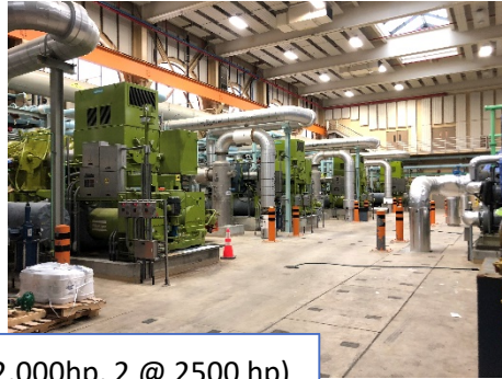
4 Large Air Compressors (2 @ 2,000hp, 2 @ 2500 hp)
