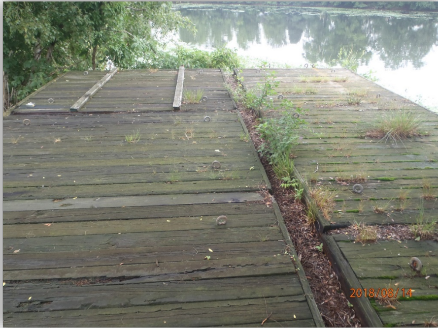
Heavy Equipment Needed to Access
