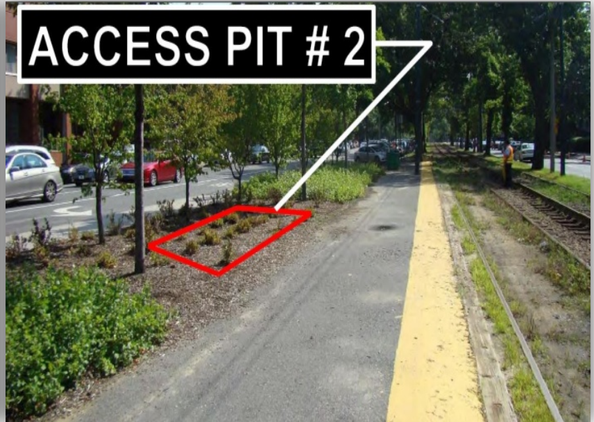
Primary Access Pit for Labor and Materials
