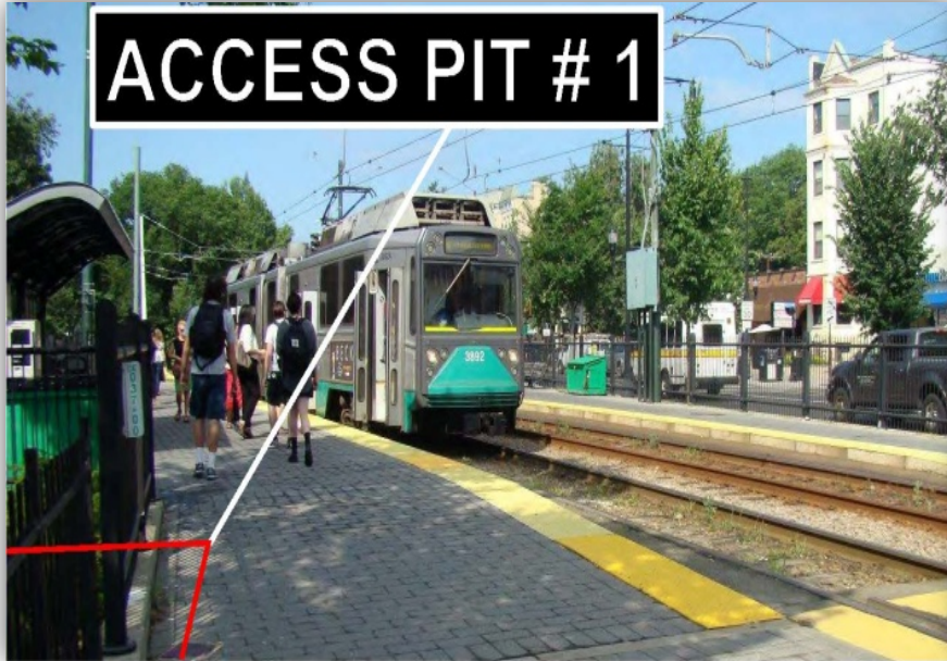
Emergency Egress Pit / Ventilation
