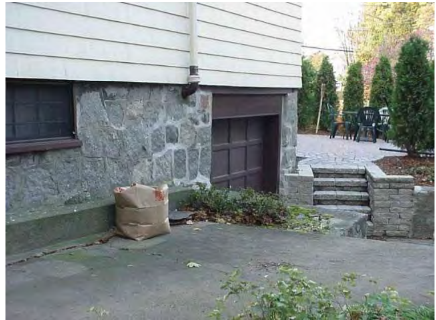
Downspout Direct Connection to Sewer
