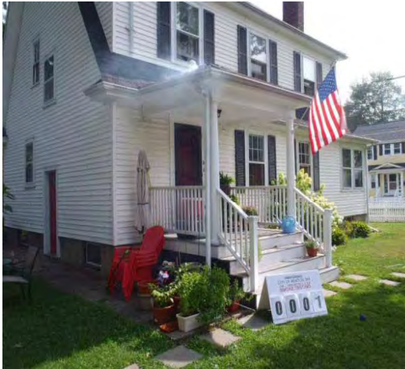
Downspout Direct Connection to Sewer
