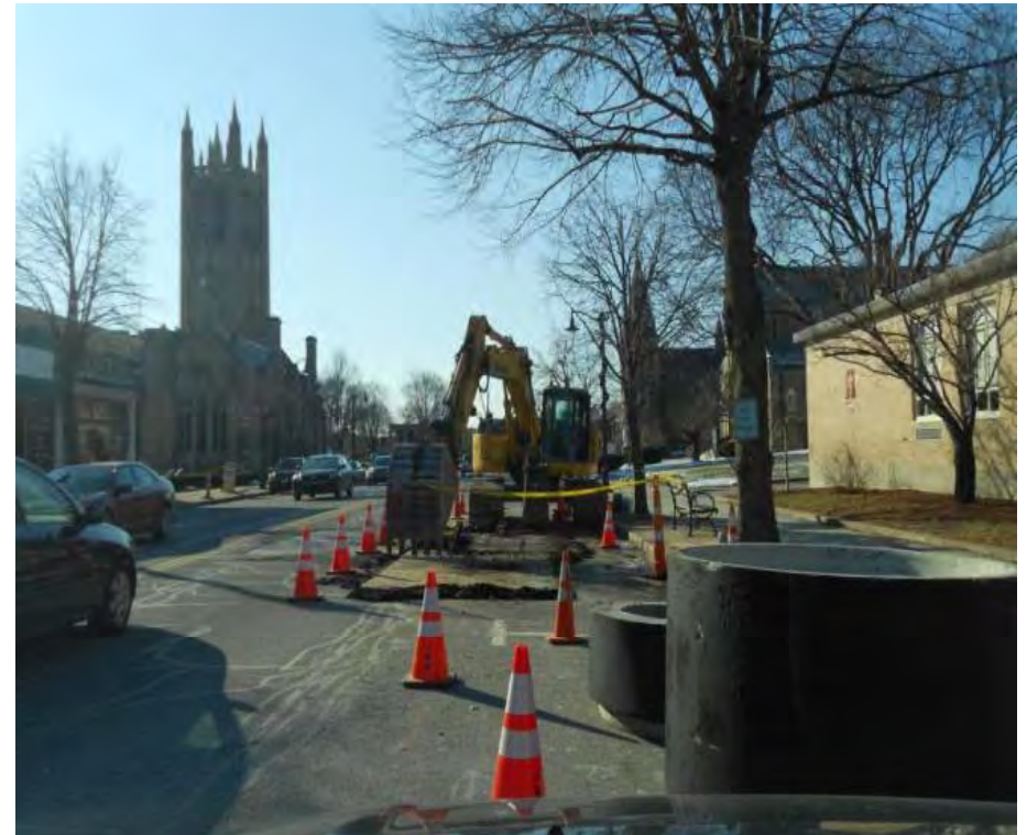
Sewer Spot Repair and New Manhole
