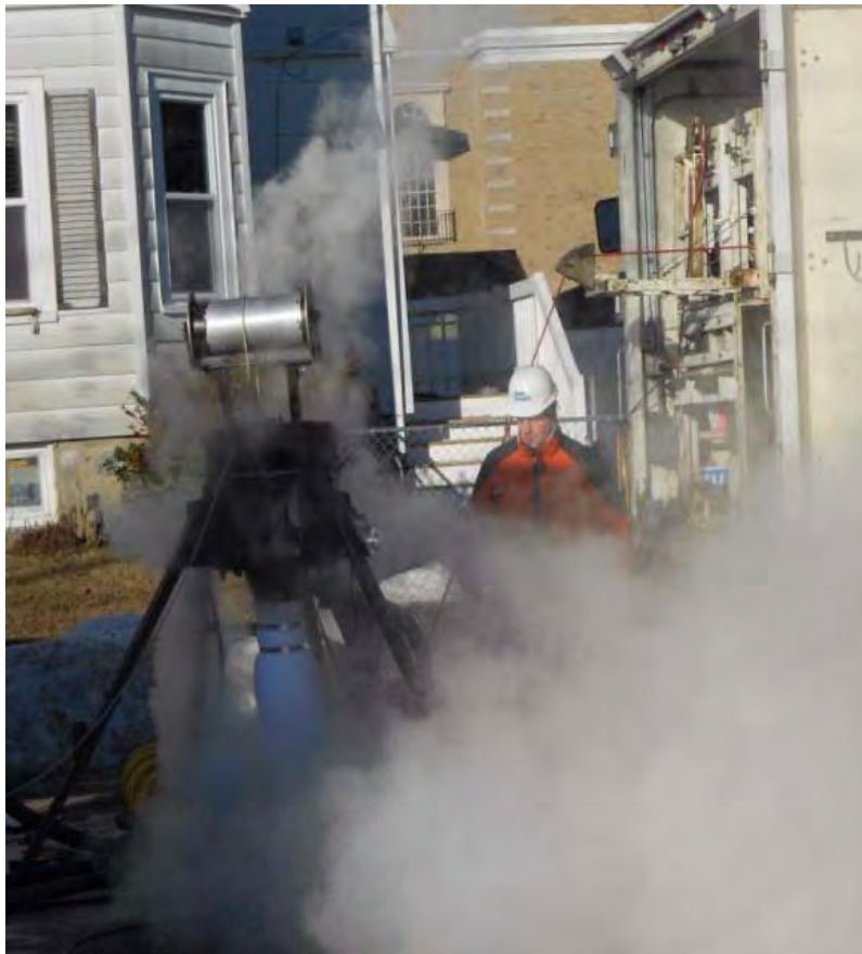
Cured-in-Place Pipe Installation
