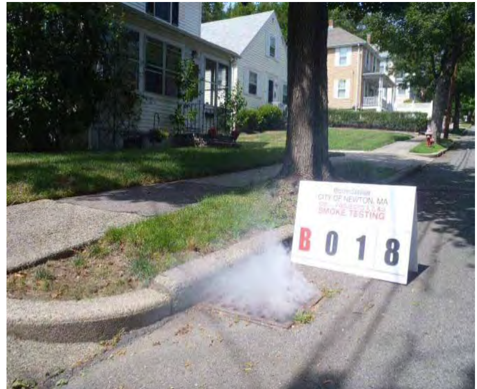
Catch Basin Direct Connection to Sewer
