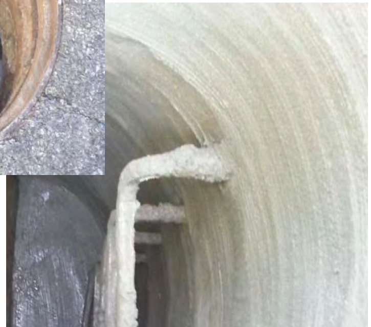
Cementitious Liner Applied
