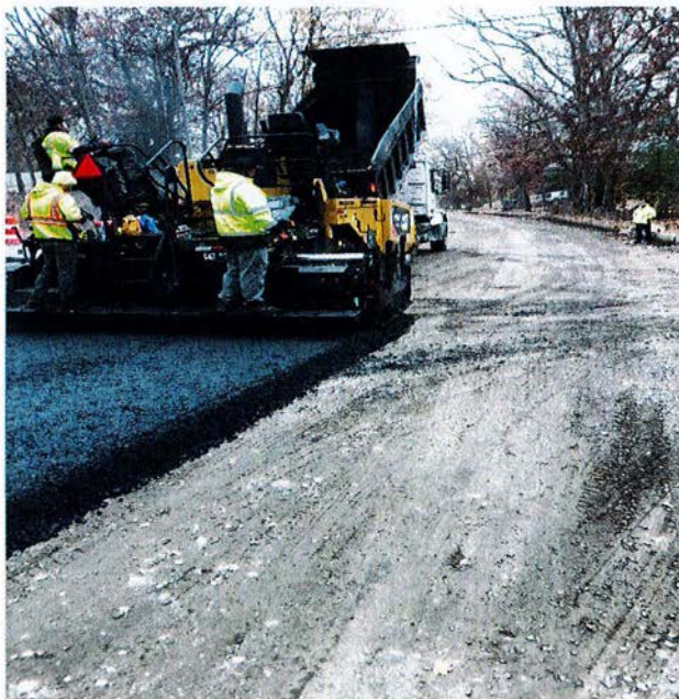
Paving after pulverization (from similar project)
