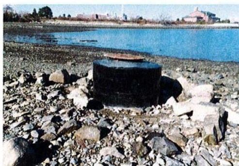
Sewer Manhole at Beach - Raised and Sealed
