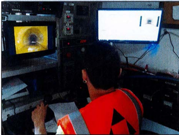
Sewer TV Inspection
