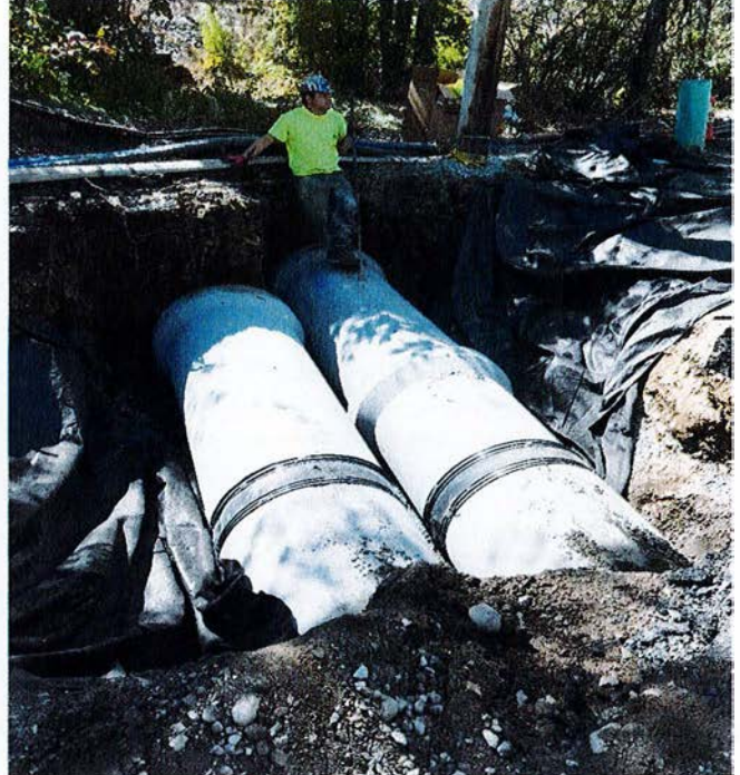
Double Barrel RCP Drain Replacement
