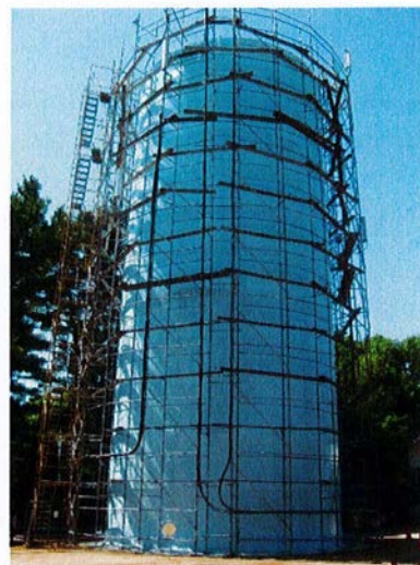
Rehabilitated Water Storage Tank
