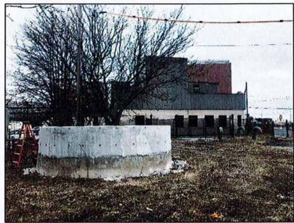
Tunnel Shaft Flood Wall
