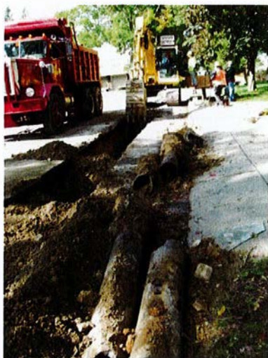
Water Main Replacement Construction
