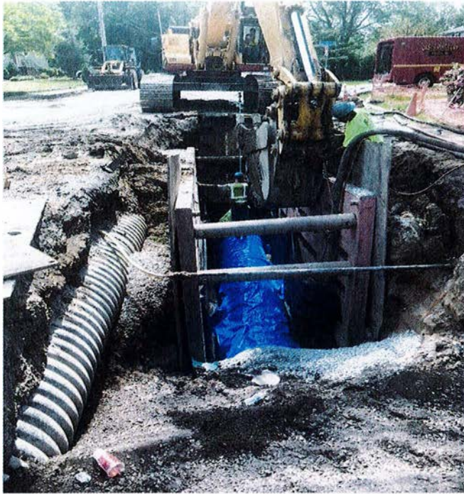
ABS Pipe Along Side New Section 111 Trench
