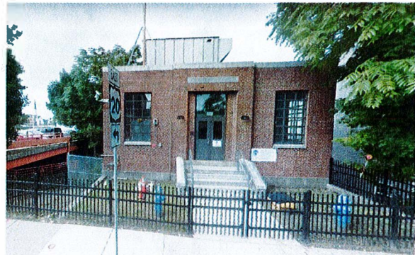
Lexington Street Pumping Station
