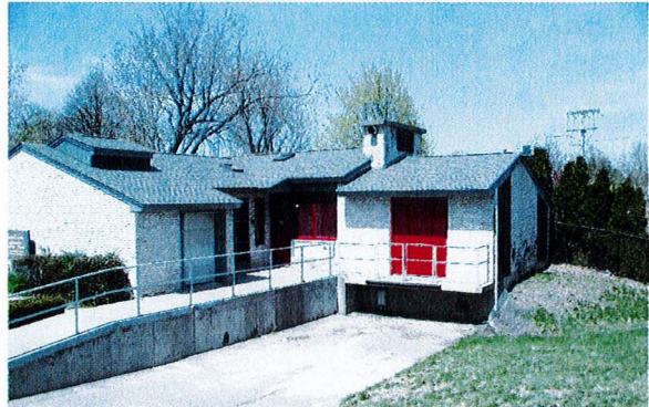
Hayes Pump Station
