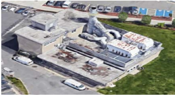
Figure 3. Ward Street Headworks
