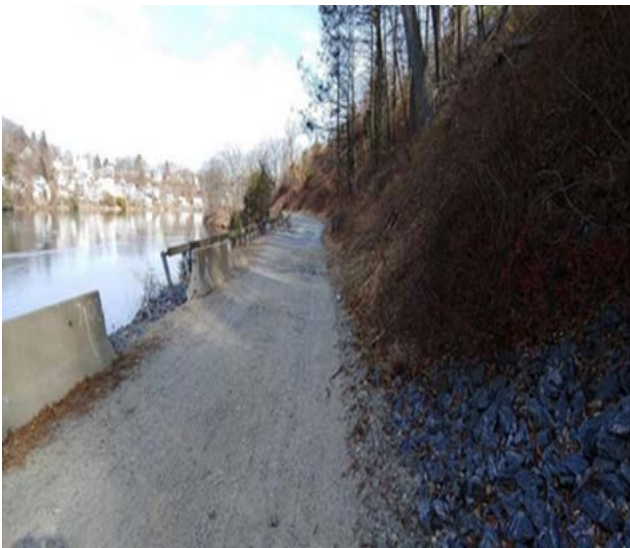
Figure 1 - River Road at Station 6+85
