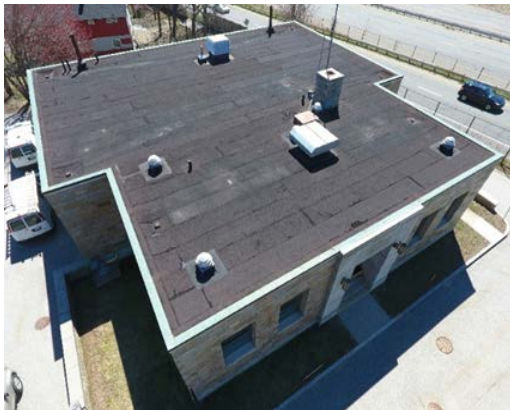
Figure 2- Spring St. Pump Station Roof
