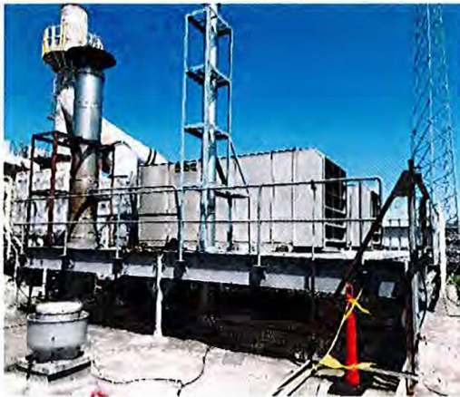
Existing dunnage framing to be demolished
