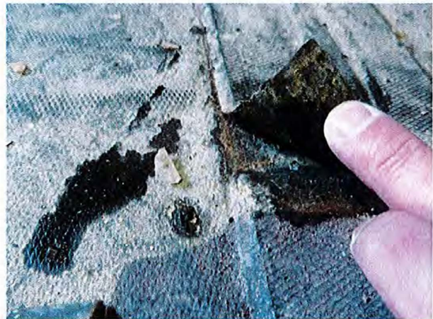
Figure 3 - Tank Lining Inspection
