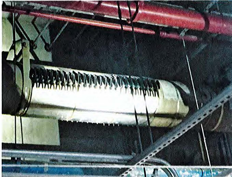
Figure 4 – Temporary Repair Sleeve
