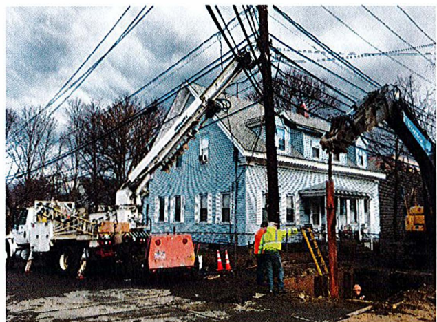
Support of telephone pole during excavation to install 30-inch drain
