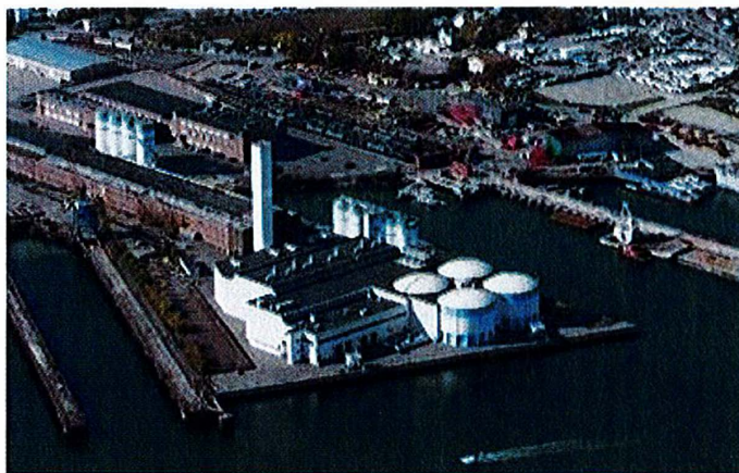
Figure 1: MWRA's Pelletizing Plant
