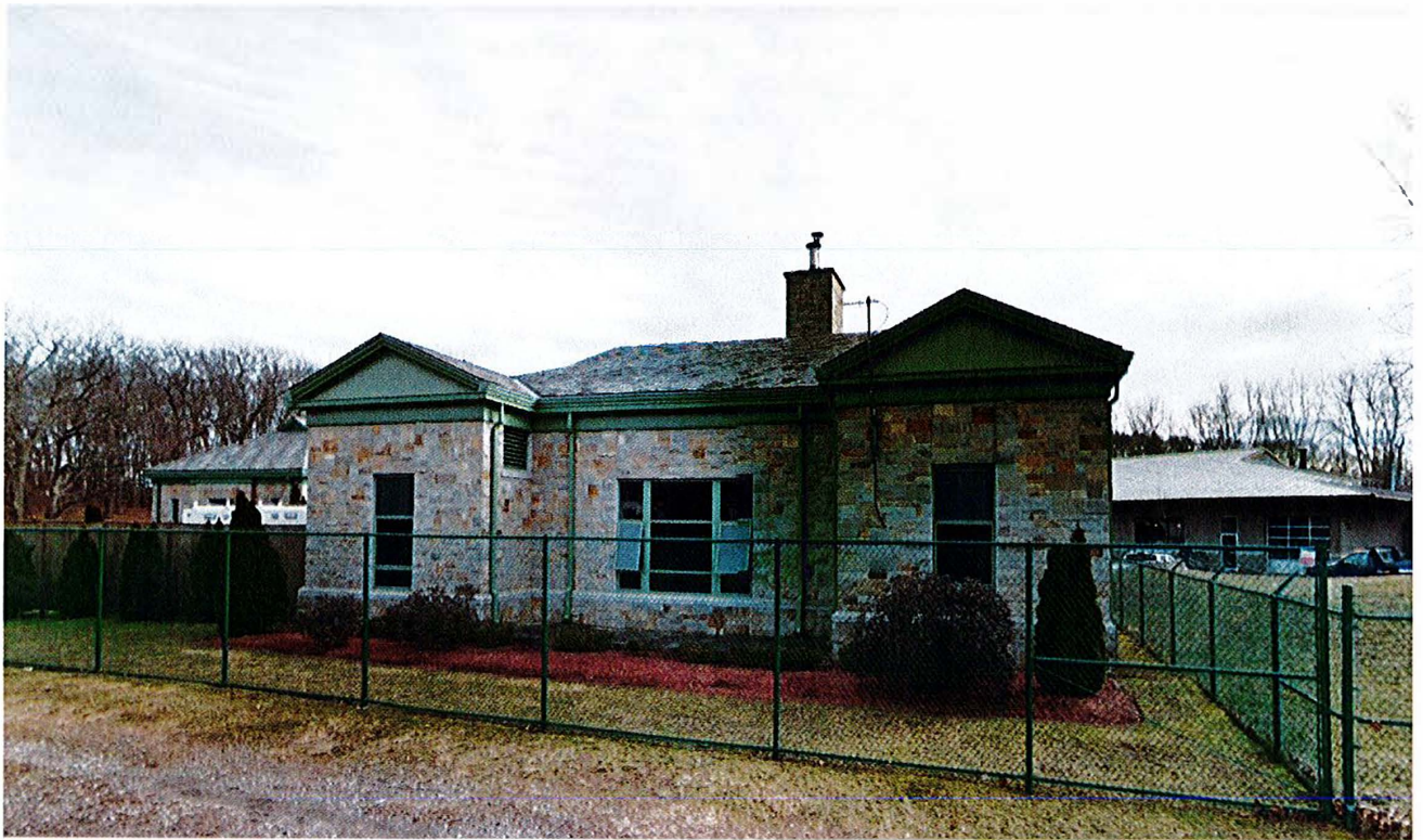
Commonwealth Avenue Pump Station, Newton
