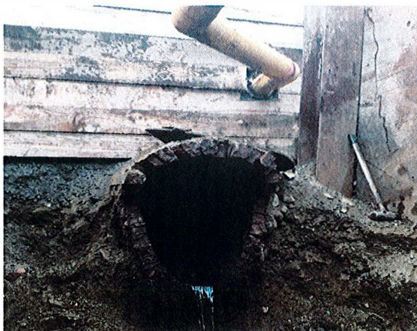
Existing drain culvert in conflict with new water line
