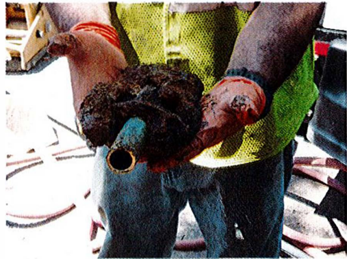
Quincy lead removal project
