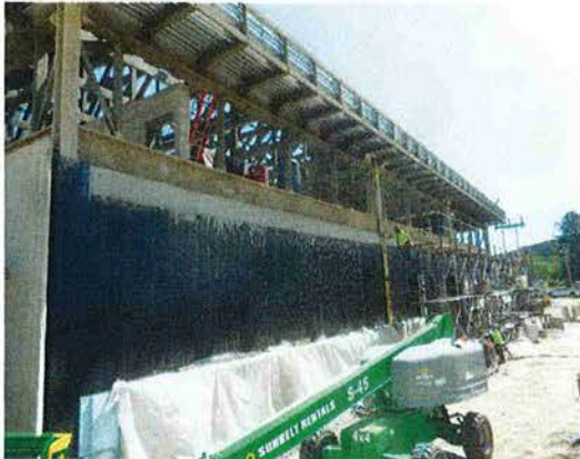
Installed bond beam
