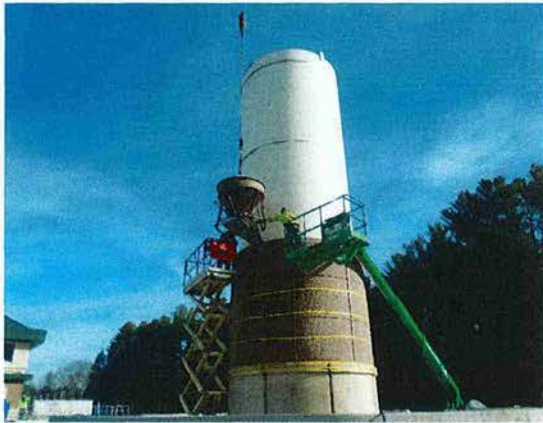
Surge Tank Construction
