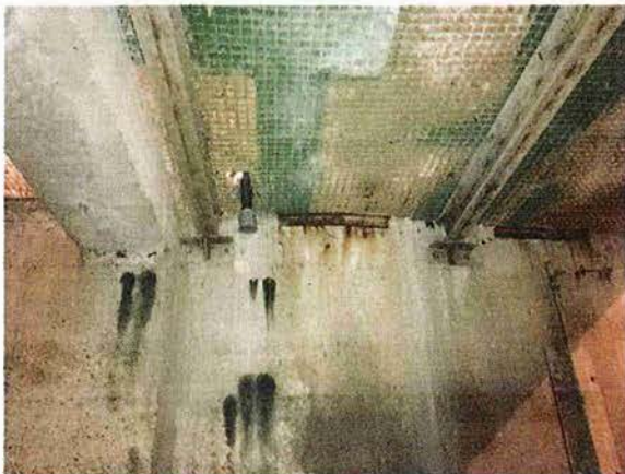
Existing anchors embedded in concrete requiring removal
