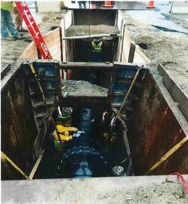
Installing 30-inch Ductile Iron Pipe in a Revised Alignment
