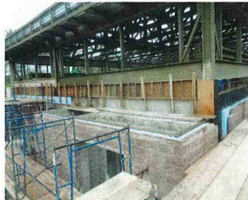
Construction of the bond beams, concrete forms and reinforcement steel
