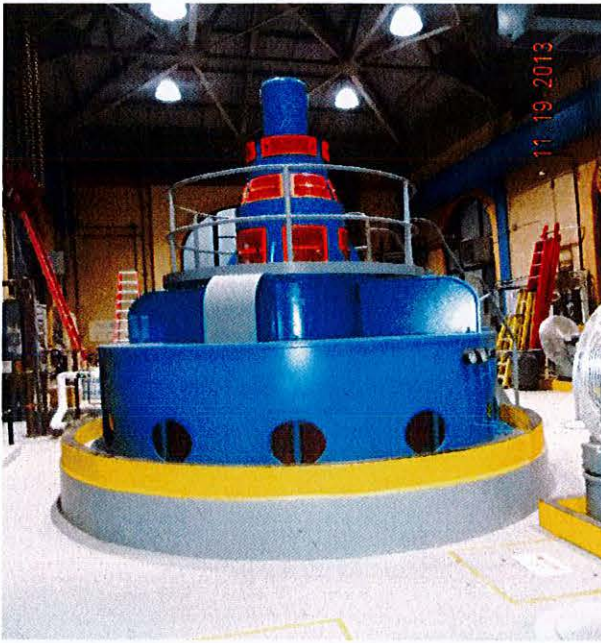
Fig. 5: Oakdale 3-MW Morgan Smith Turbine
