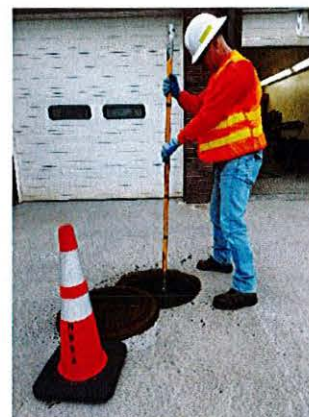
Figure 2. Inspection of a gas/oil separator.
