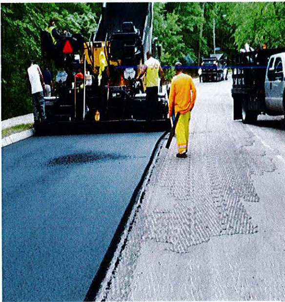
Full width mill and overlay on Enneking Parkway
