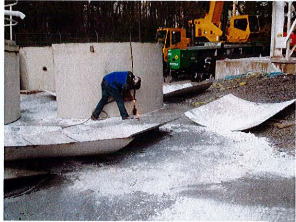
Cutting silo tanks in place
