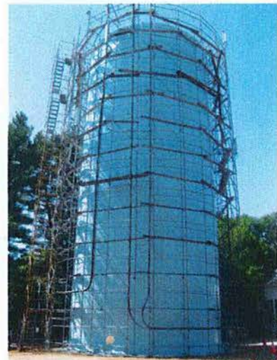
Rehabilitated Water Storage Tank
