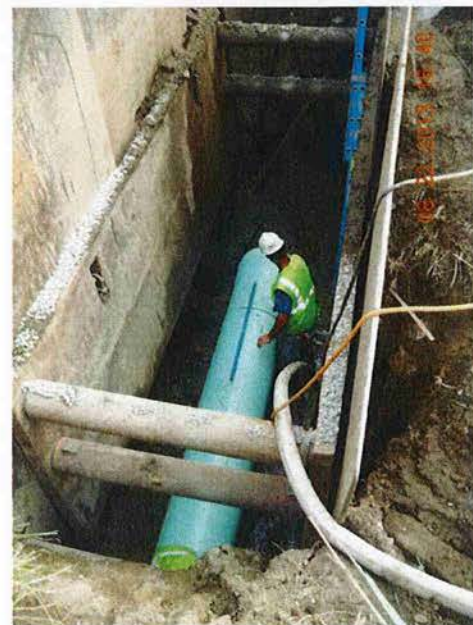
Installation of New PVC Sewer Pipe
