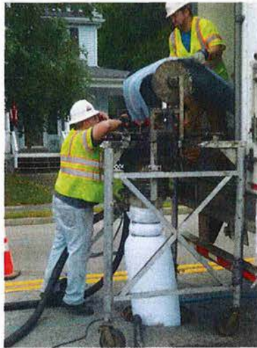
Installation of Cured-In-Place-Pipe Liner
