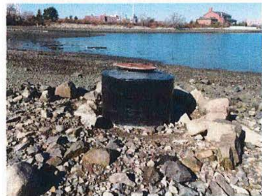
Sewer Manhole at Beach - Raised and Sealed
