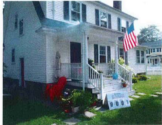
Smoke Testing Confirms House Downspout is an Inflow Source Connected to the Sewer
