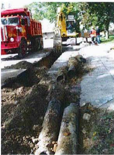
Water Main Replacement Construction
