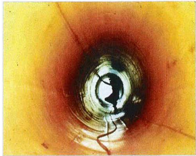
Cured-In-Place-Pipe Liner
