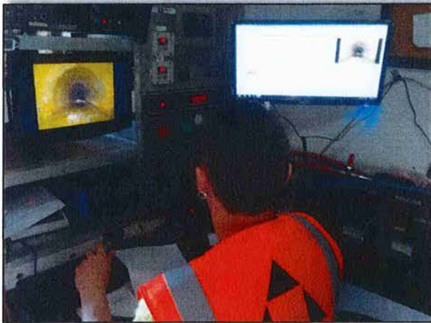
Sewer TV Inspection
