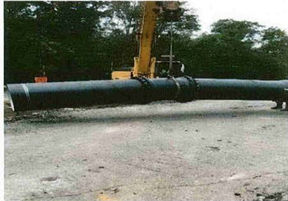
Installation of 11 ¼ Degree Bend at 23+44
