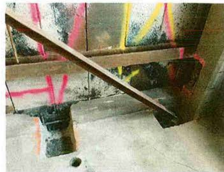
Chipping PCB concrete to expose structural steel
