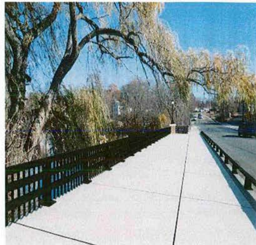
Section 111 Pipeline Crossing Mother Brook
