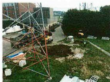
Removal of PCB Contaminated Soil
