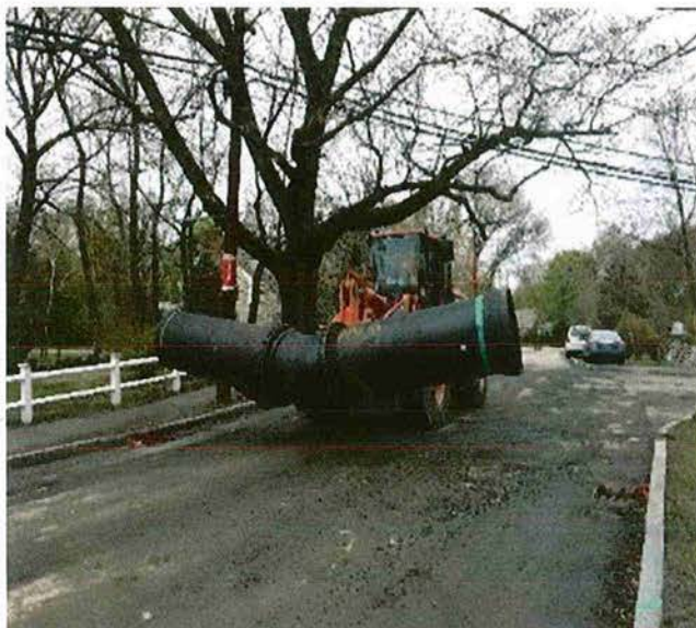
Hopkins Street, Reading – Transporting 36-inch restrained joint bend for installation
