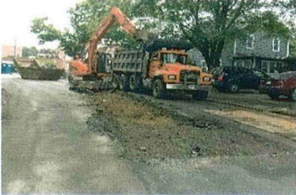
North Street – Stoneham Removing asphalt prior to installation of 48-inch
