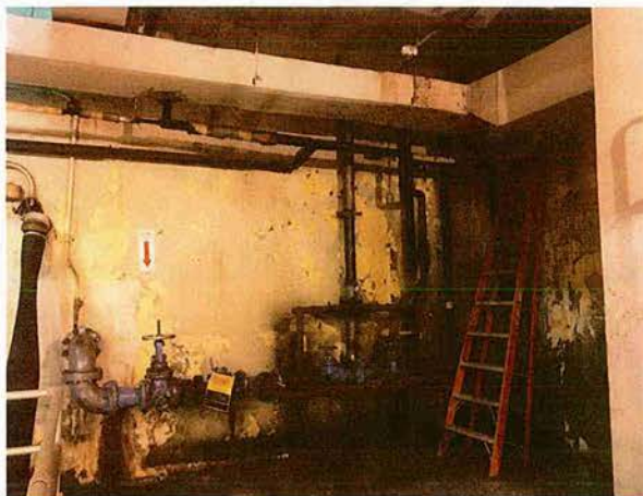
Existing water service piping
