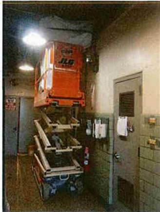
Mini-containment for PCB coring
