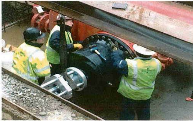
Section 77 tapping machine being mounted
