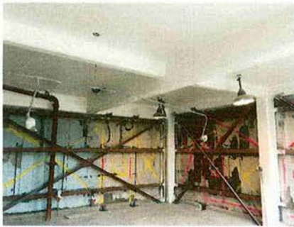
Girt framing modifications
