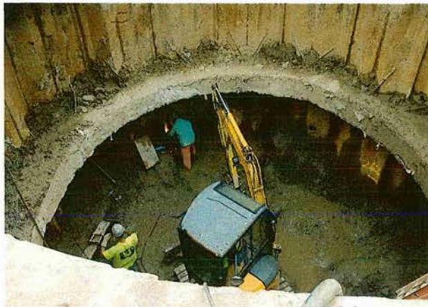
Excavation for the Surge Tank
