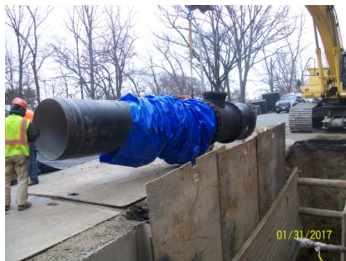
Typical 36" pipe being installed.
