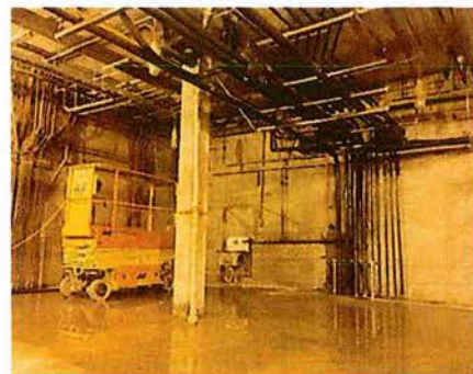
Abatement of PCB Paint in Mezzanine Level (After)
