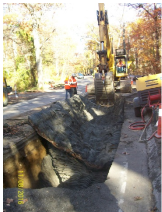
Typical blasting mat being removed.
