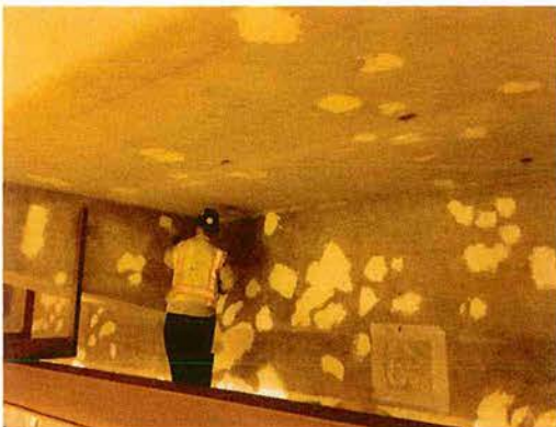
Trowel applied epoxy resurfacer to seal imperfections in the porous surfaces
