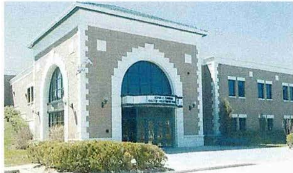
John J Carroll Water Treatment Plant
