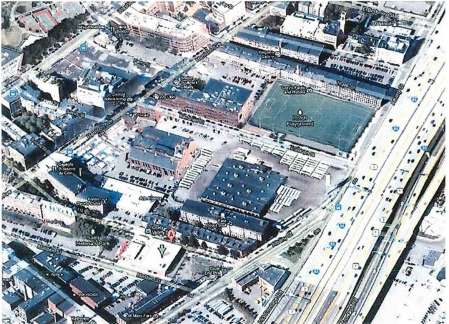
Aerial Map of Union Park Pump Station/CSO Facility
