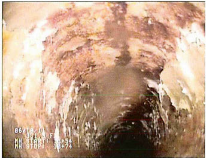
Figure 1 - CCTV Photo of Section 4
