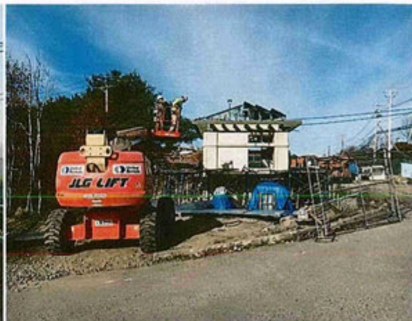
Construction progress of the new Guardshack
