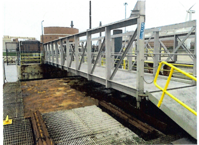
View from floating dock no. 1 of the gangway
