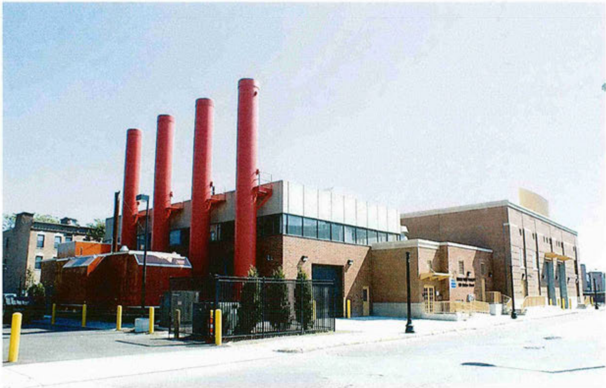
Union Park Pump Station/CSO Facility
