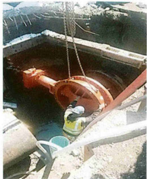
Installation of a 48" Butterfly Valve
