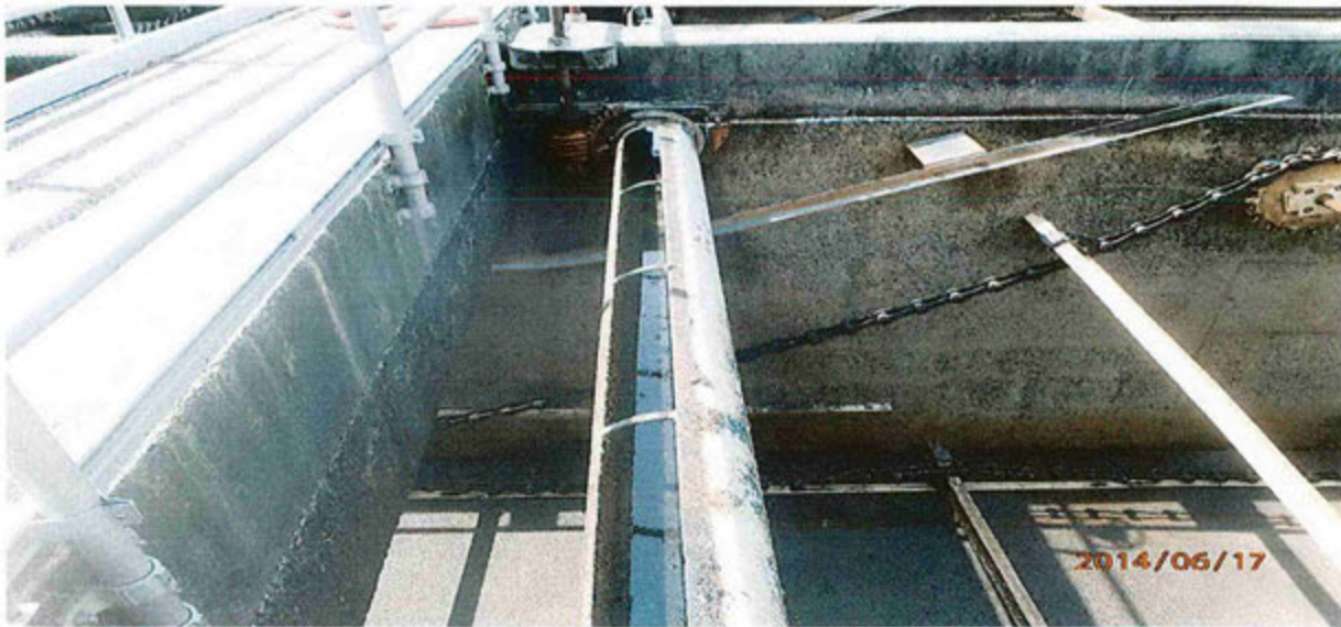
Clinton Wastewater Treatment Plant Clarifier Upgrades (Pre-Construction)
