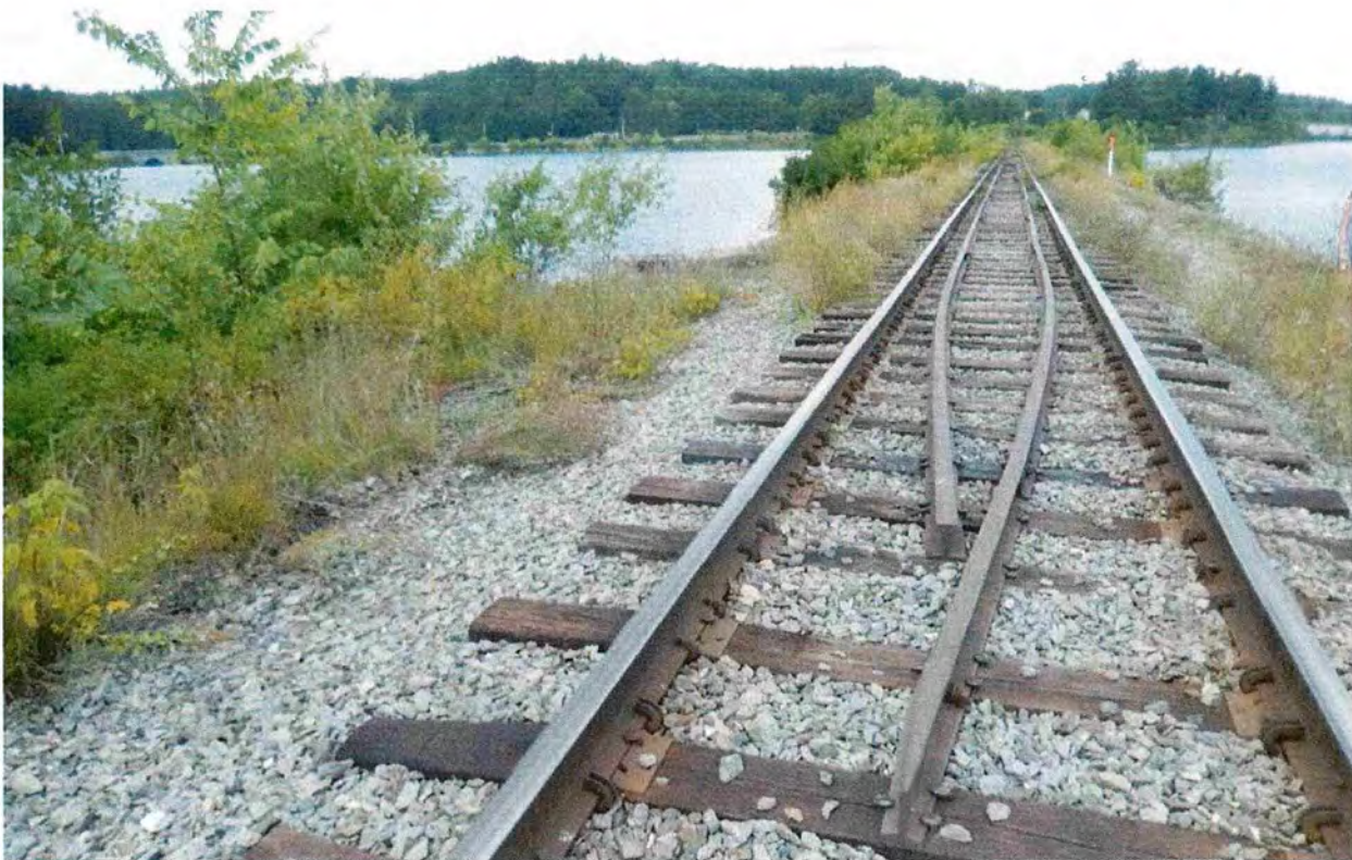
Guard Rails Installed by PanAm Railway at Quinapoxet Causeway
