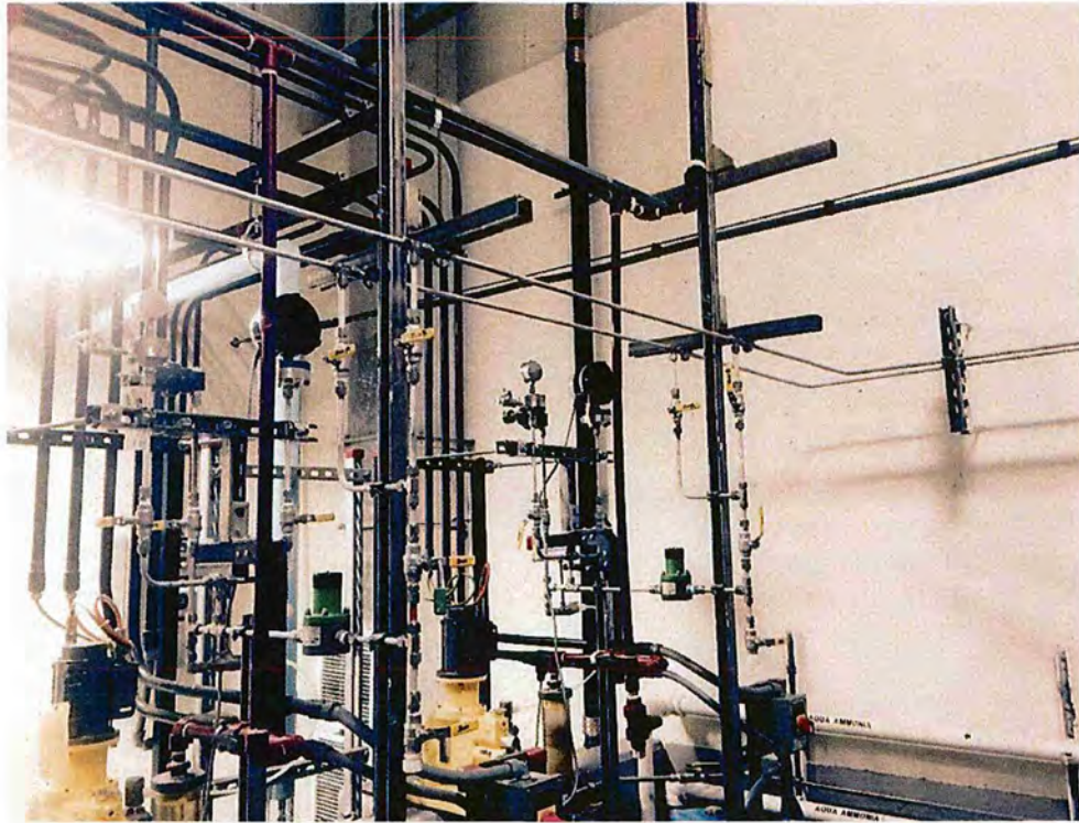
Carroll Treatment Plant ammonia system piping improvements
