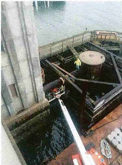
Leak Repairs near North Tunnel Shaft, 2014
