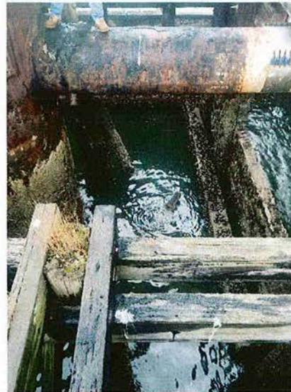
Leak Repairs - Welded Plug & Mechanical Clamp
