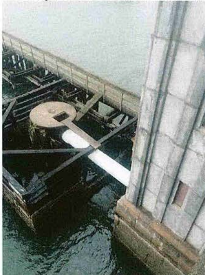
Corrosion Protection at South Tunnel Shaft
