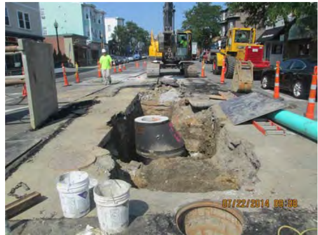
12-inch Storm Drain Installation on East Broadway Reserved Channel Sewer Separation Contract 4
