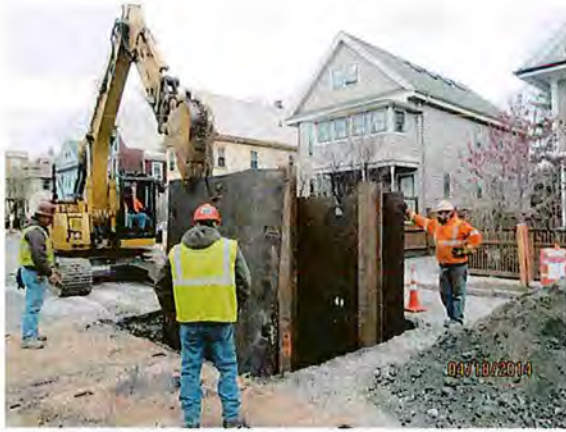
Sheeting for Drain MH on Concord Avenue Cambridge Sewer Separation Contract 9
