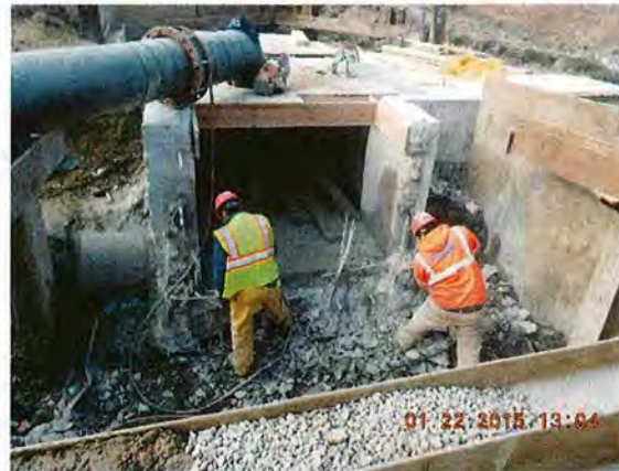
Modifications to CSO Regulator Structure RE031 at Outfall MWR003
