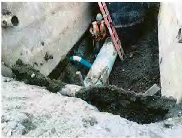
Reservoir Street 18-inch Sewer Installation CAM004 Sewer Separation Contract 8B
