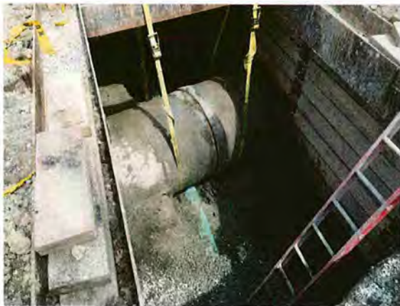
Reservoir Street 18-inch Sewer Installation CAM004 Sewer Separation Contract 8B
