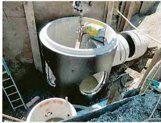
Concord Avenue Drain Installation Cambridge Sewer Separation Contract 9
