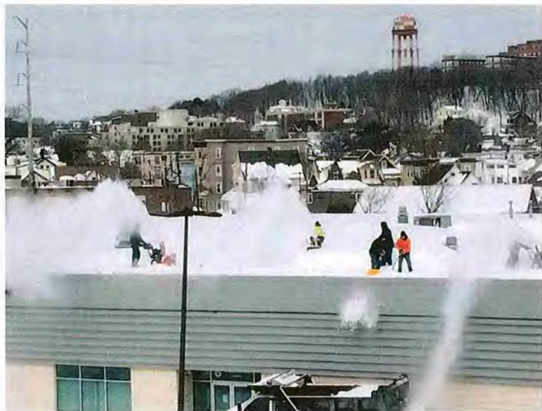
MWRA Staff Clearing Snow from Chelsea Facility Roof
