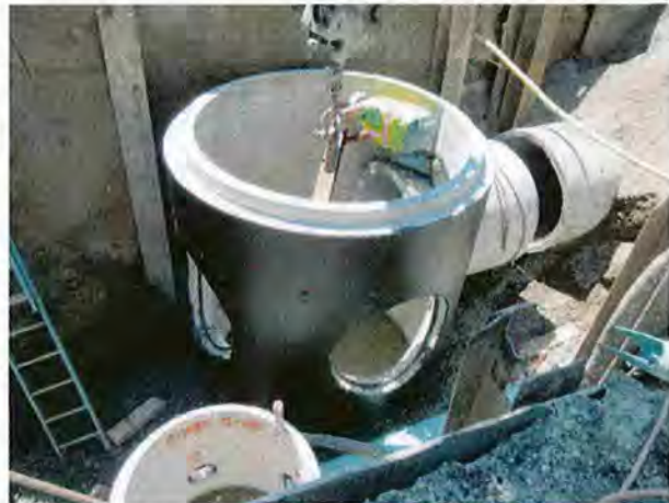
Concord Avenue Drain Installation Cambridge Sewer Separation Contract 9
