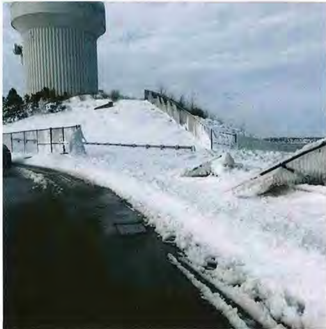
Damaged Perimeter Security Fence At Deer Island
