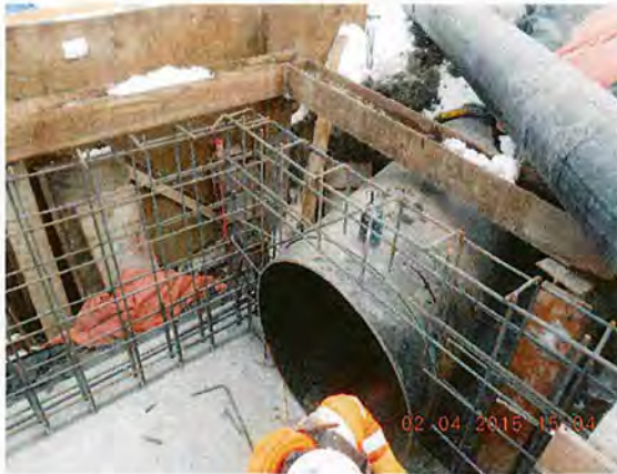
48-Inch Diameter Replacement Siphon at Outfall MWR003
