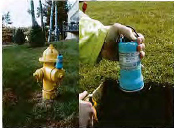
Correlation survey accelerometer (datalogger) and placed on a hydrant
