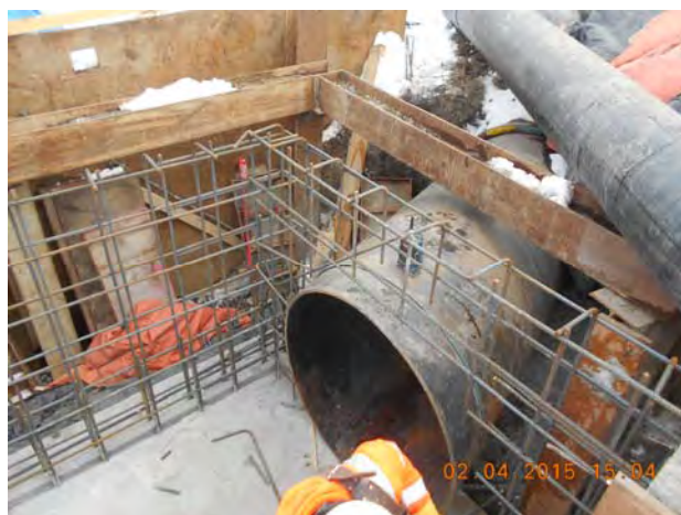
48-Inch Replacement Siphon at Outfall MWR003
