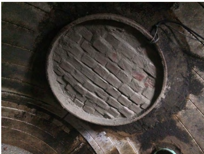
Brick and mortar bulkhead of high outlet overflow in CSO regulator CHE002-3.
