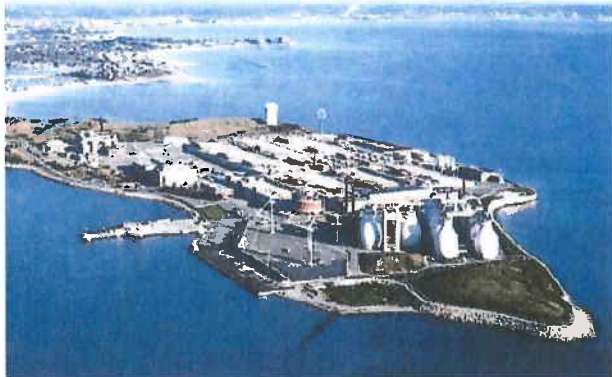
Deer Island Treatment Plant
