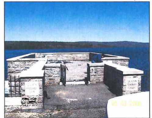
Chicopee Valley Aqueduct Intake Building
