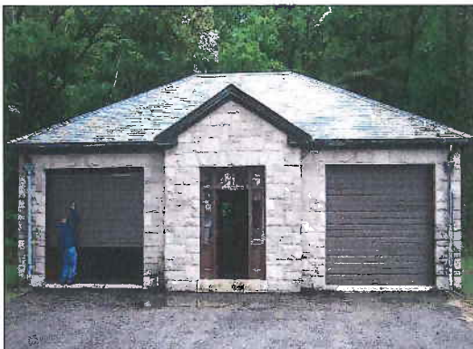
Quabbin Aqueduct Shaft 12 Service Building
