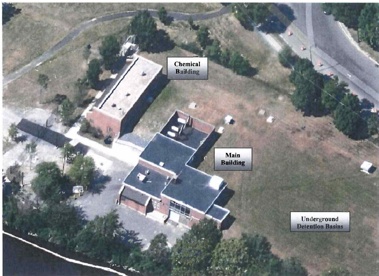
Figure 1: Cottage Farm Facilities
