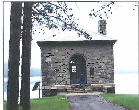
Quabbin Aqueduct Shaft 12 Intake Building
