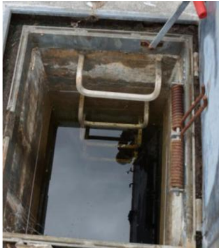
Shaft 7D chamber
