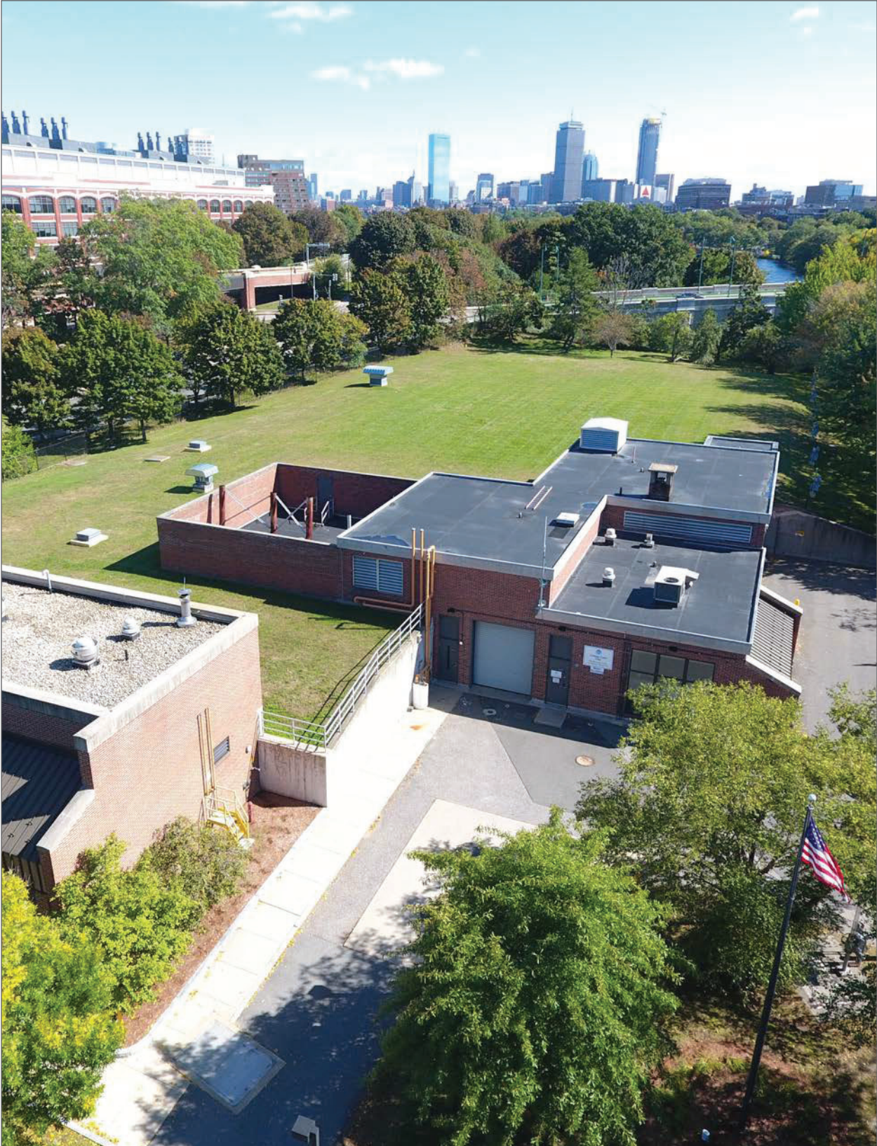
Cottage Farm CSO Facility, Cambridge
