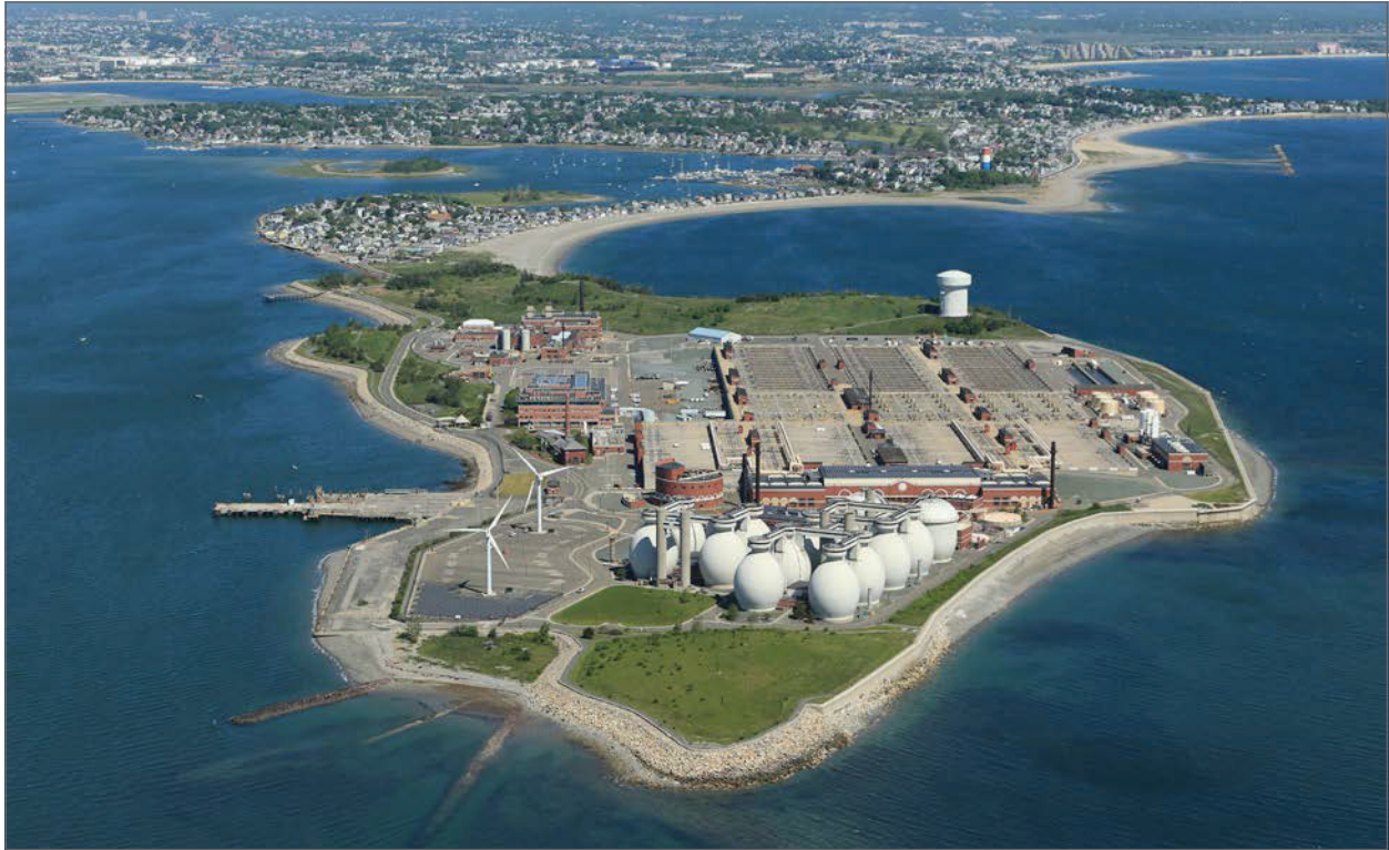
Deer Island Wastewater Treatment Plant
