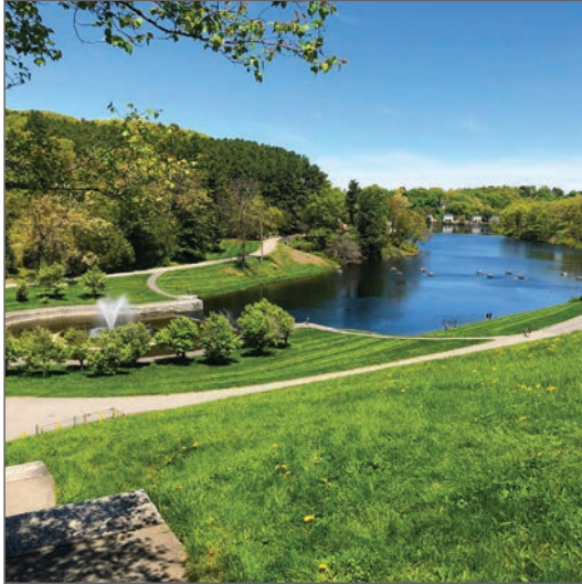
Backside of the Wachusett Dam
