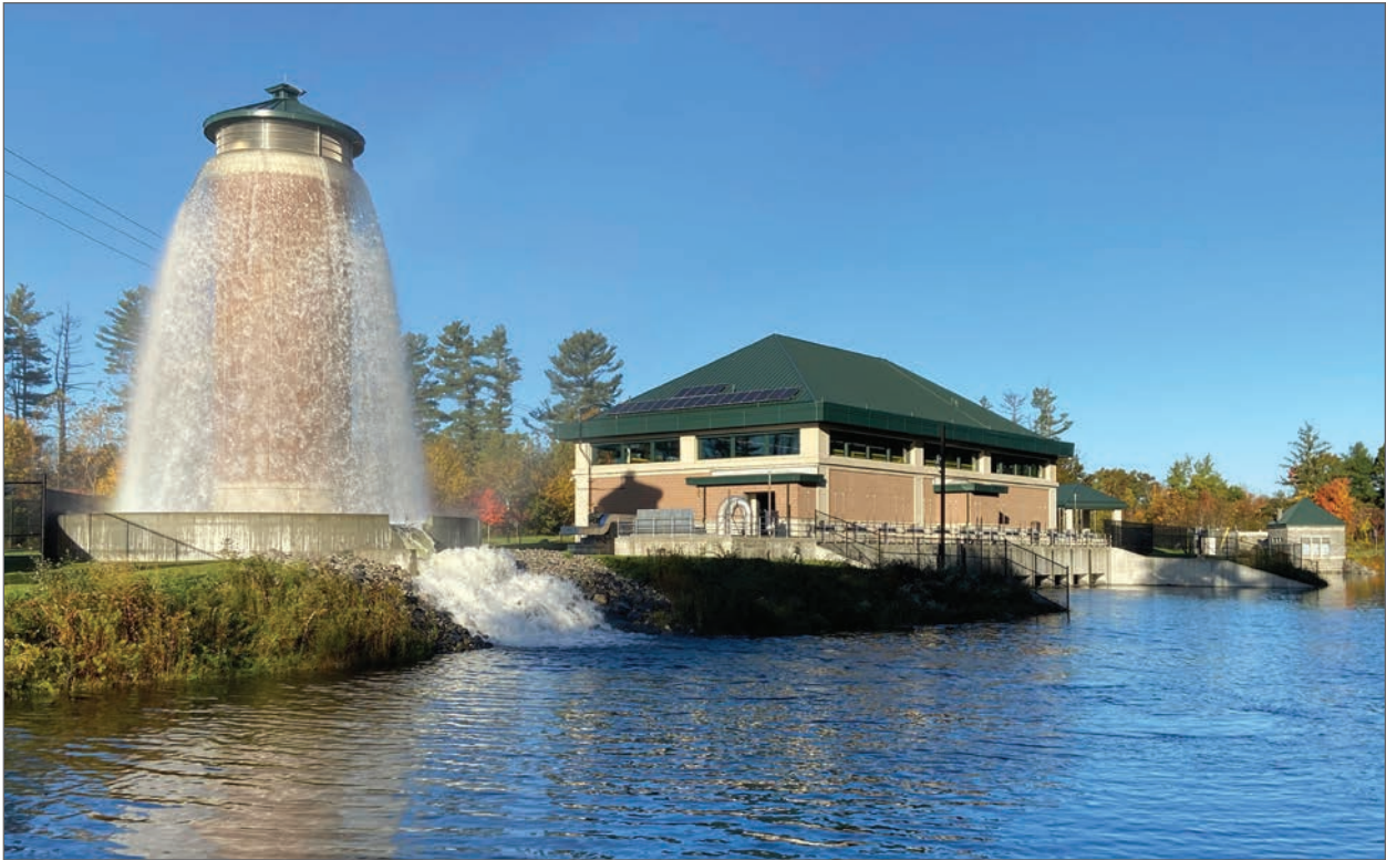
Wachusett Aqueduct Pumping Station
