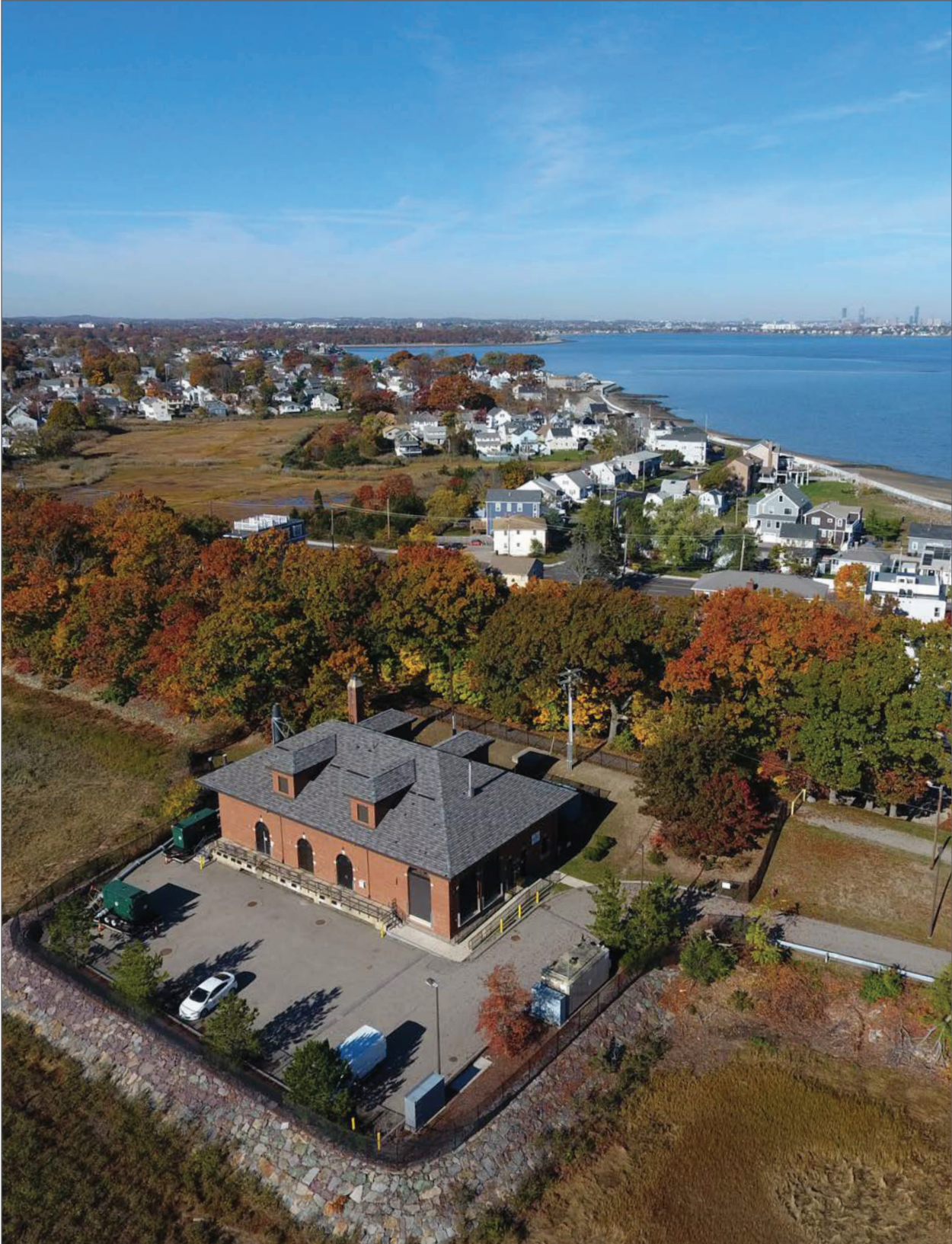
Braintree-Weymouth Pump Station, Quincy
