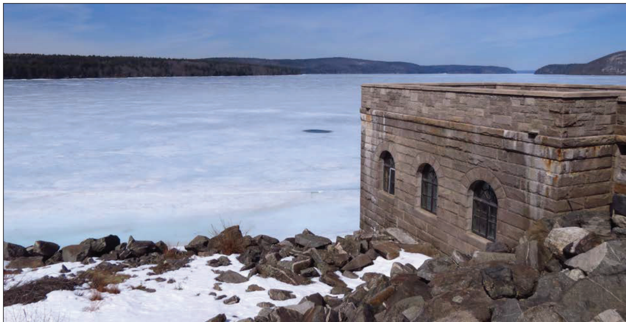
Winsor Dam Intake at Quabbin Reservoir
