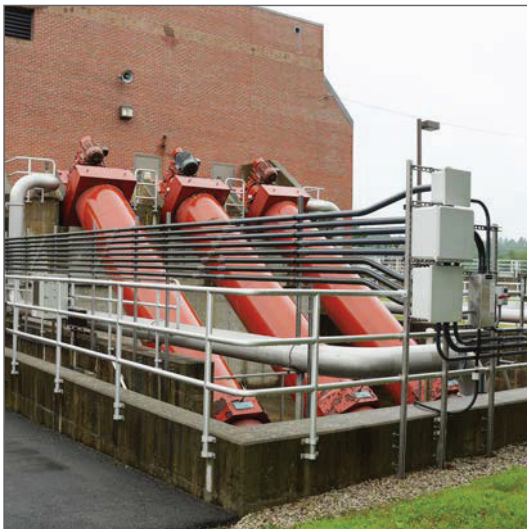
Clinton Wastewater Treatment Plant
