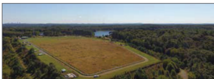
Norumbega Covered Storage Facility in Weston
