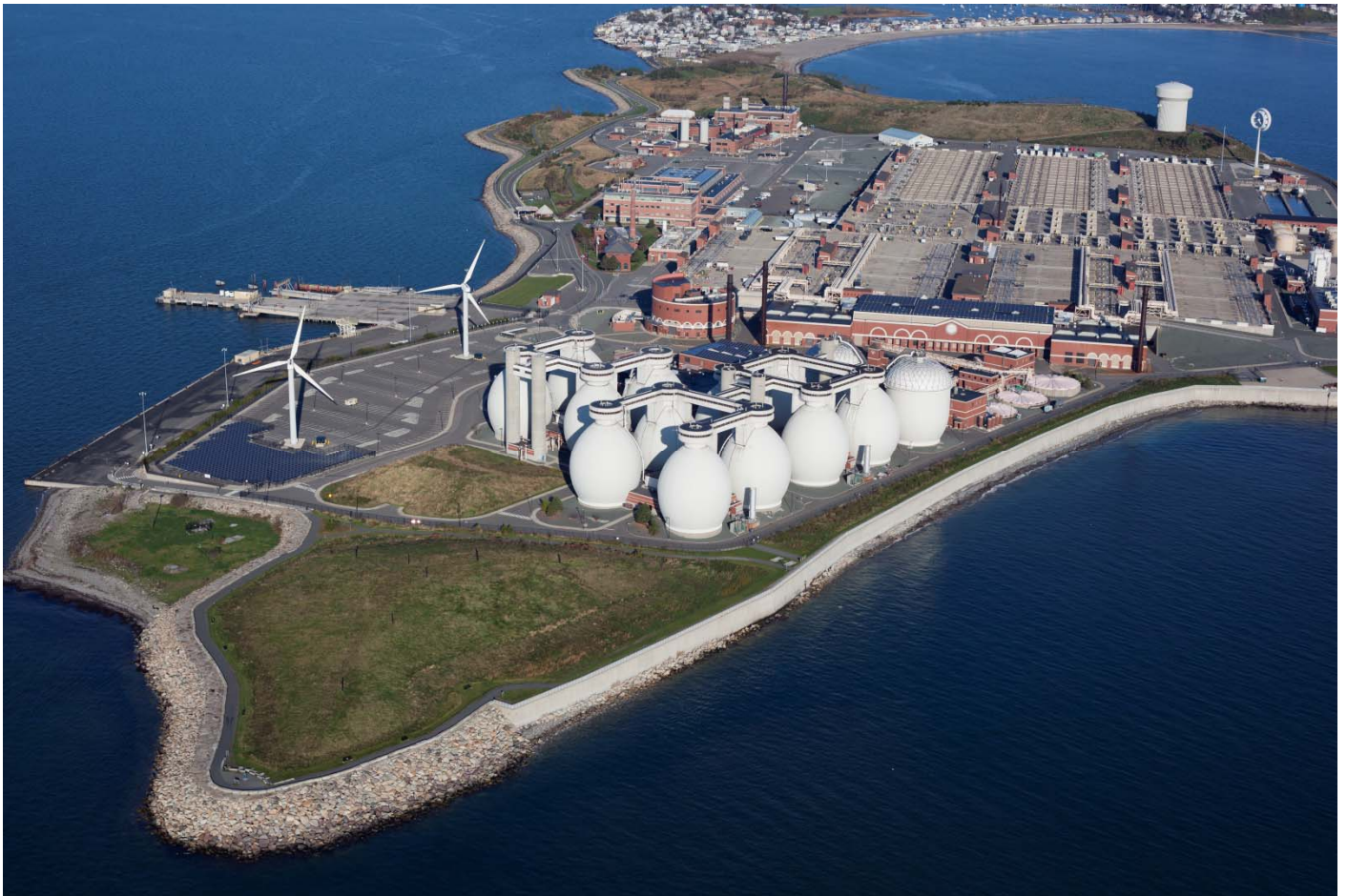
Deer Island Wastewater Treatment Plan
