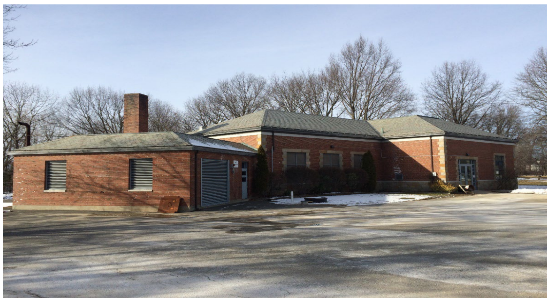
Alewife Brook Wastewater Pump Station
