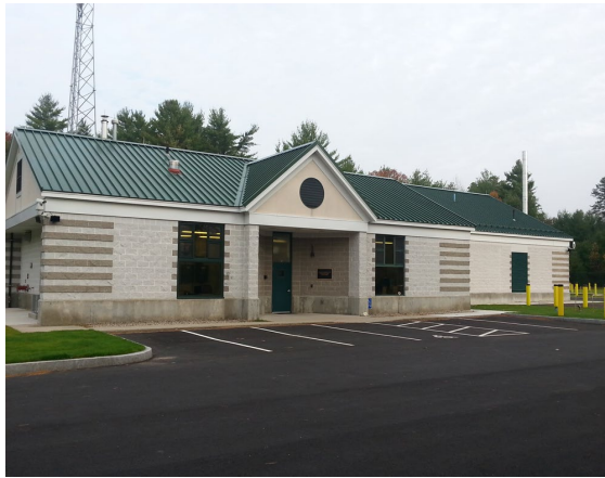
Brutsch Water Treatment Facility
