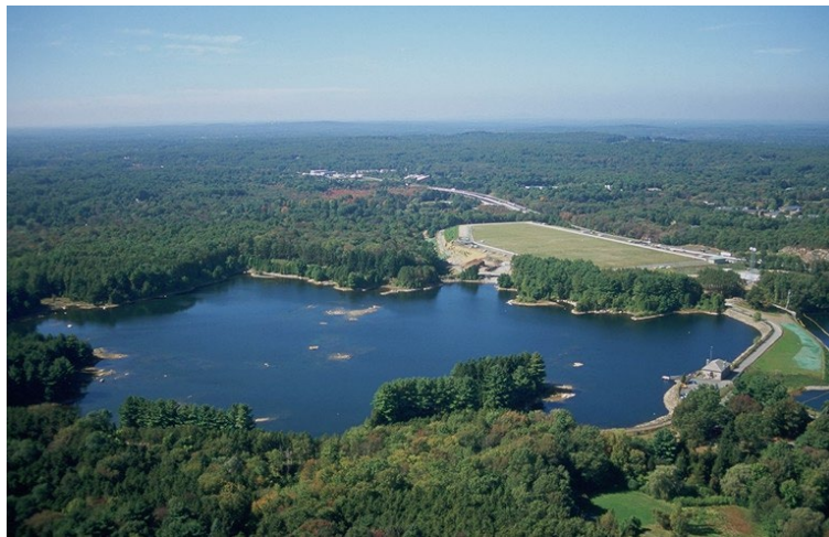
Norumbega Covered Storage Tank and Norumbega Open Reservoir (now a backup supply)
