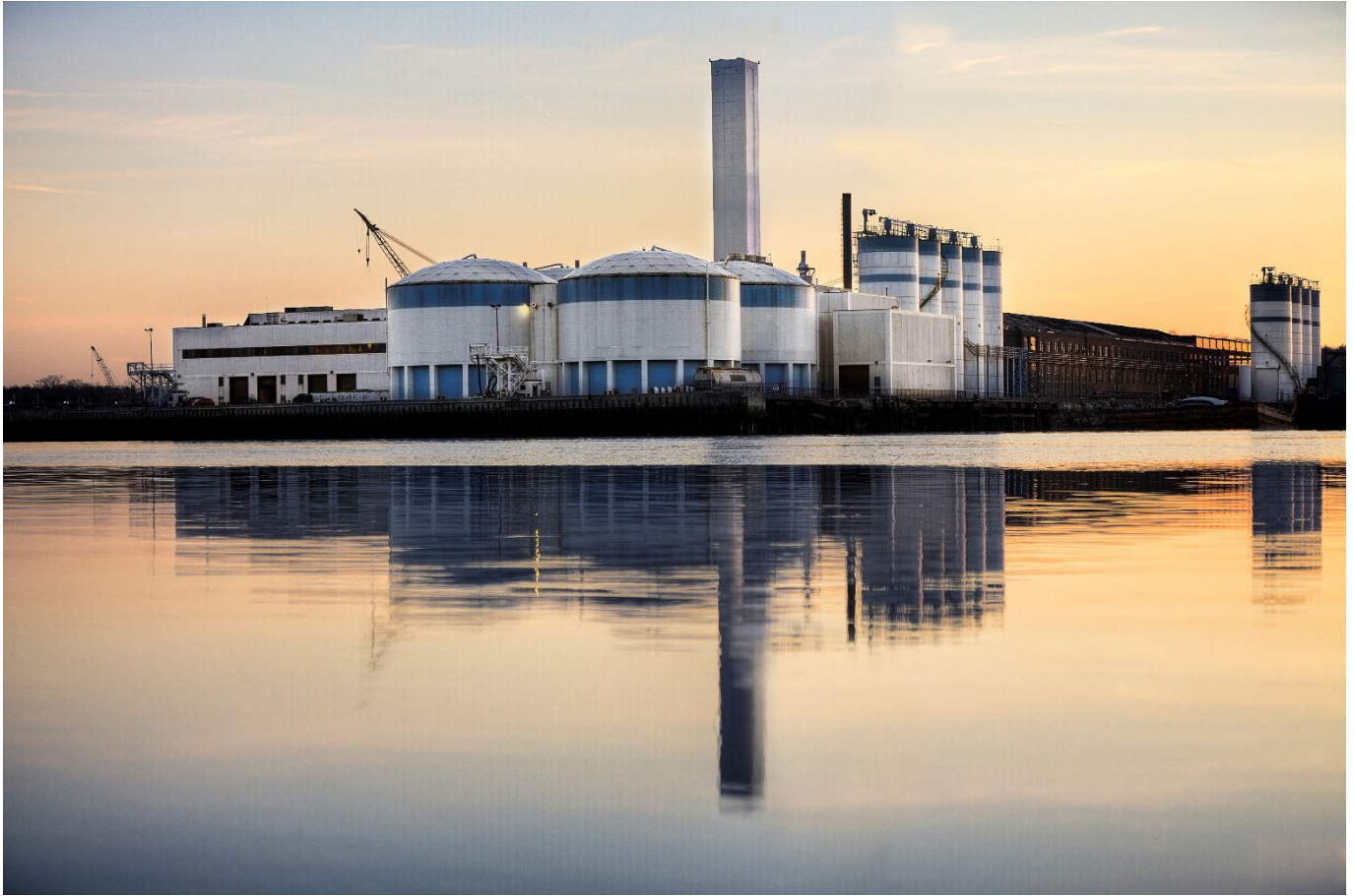
MWRA Sludge Pelletizing Facility
