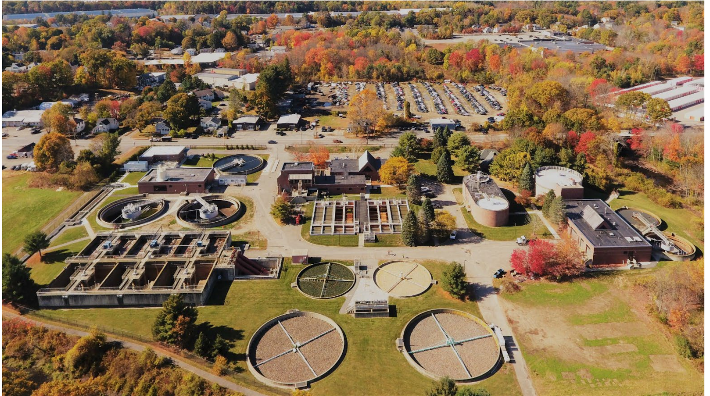
Clinton Wastewater Treatment Plant
