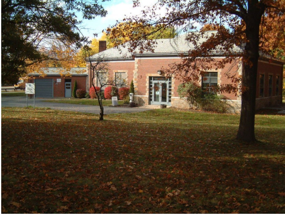
Alewife Brook Wastewater Pump Station
