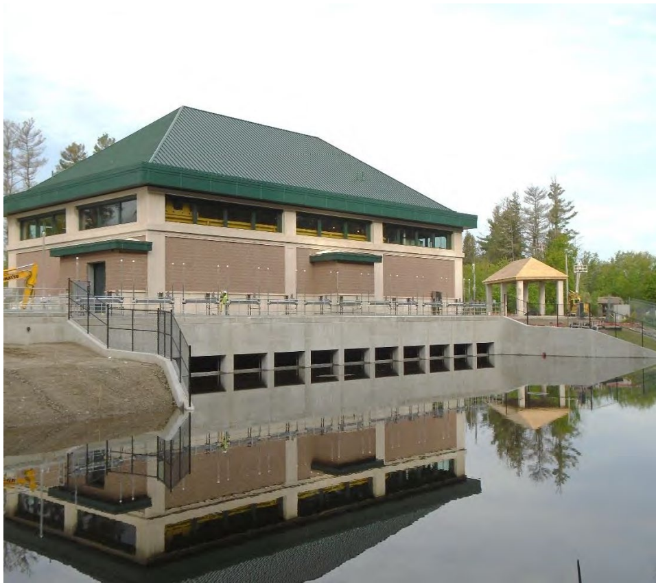
Wachusett Aqueduct Water Pump Station Forebay
