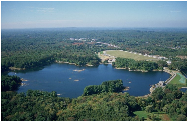
Norumbega Covered Storage Tank and Norumbega Open Reservoir (now a backup supply)
