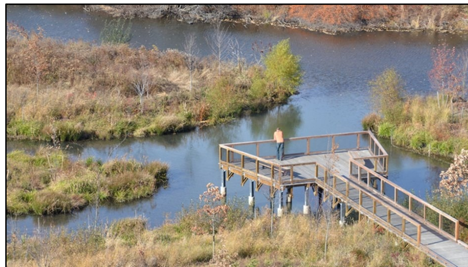
Stormwater Wetland to Manage Separated Stormwater Flows
