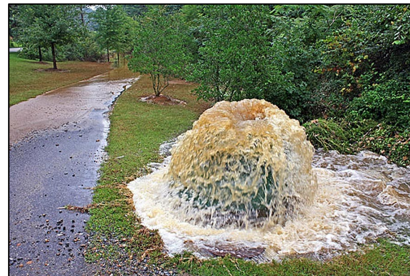
Sanitary Sewer Overflow
