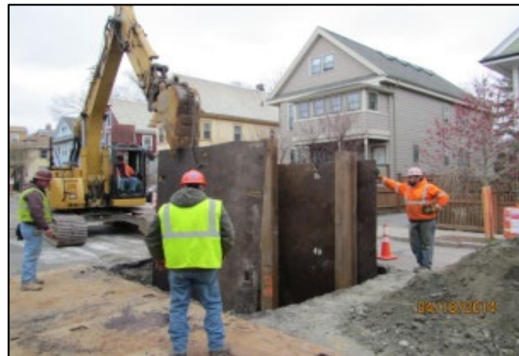
Sewer Separation on Concord Ave, Cambridge
