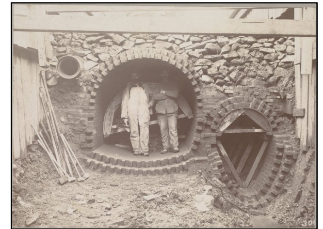
Construction of Metropolitan Sewer District combined sewers, 1880s
