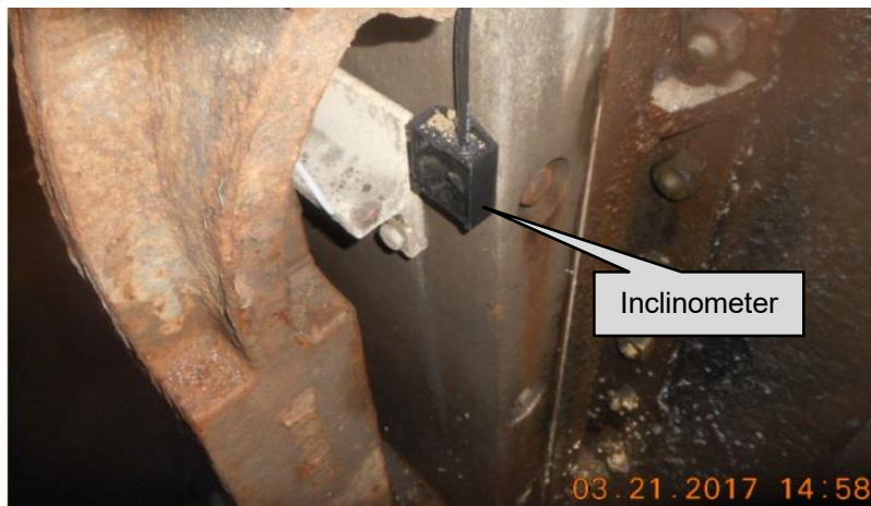
Figure 7-3. Inclinometer Installed on a Tide Gate
