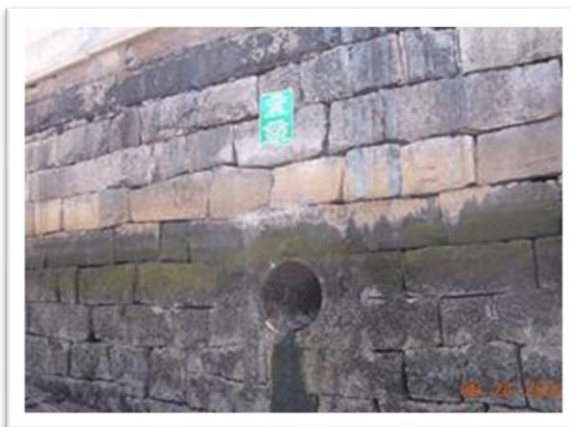
Former CSO Outfall CHE002 now discharges only stormwater
