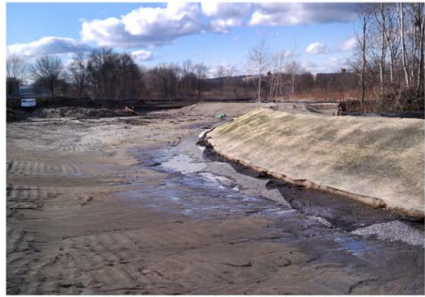
Perimeter Berm at Future Wetland Basin
