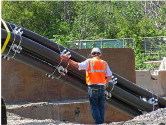
Launching Electric Bundle into Pit
