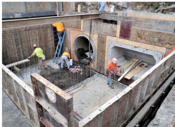
Stormwater Diversion Structure
