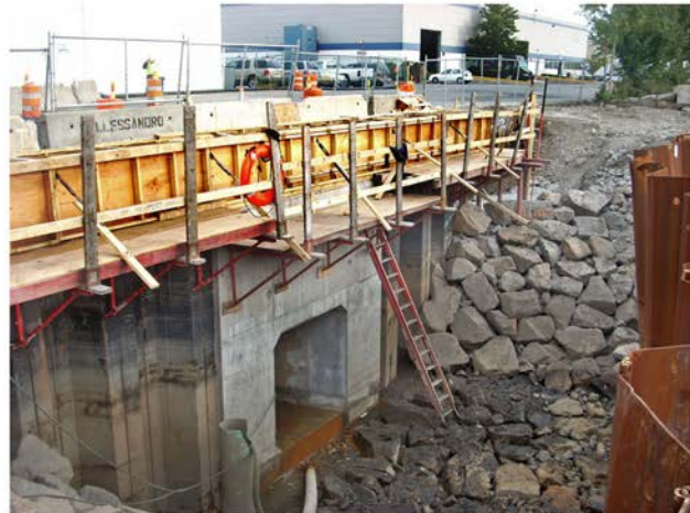
Bridge guard rail and outfall headwall construction on Papas Way
