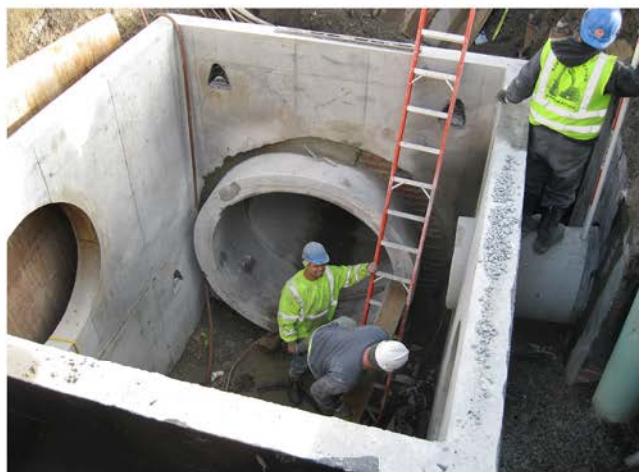
Installation of Special Manhole C at West First Street and F Street
