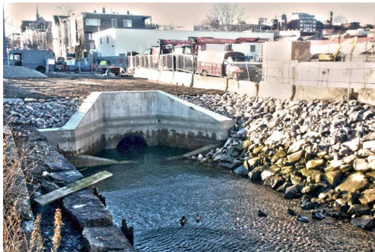
Completed Rehabilitation of Outfall BOS078
