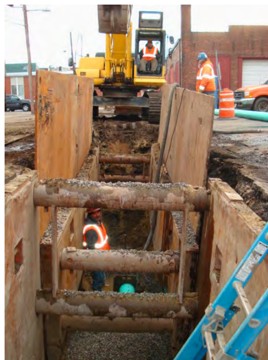
New sewer installation along Whittemore Avenue in Cambridge
