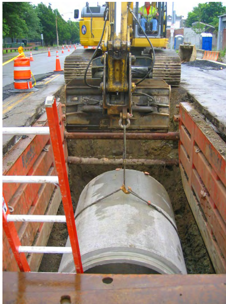
66" drain installation in Farragut Rd.
