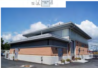
North Dorchester Bay CSO Storage Tunnel Dewatering Pump Station, Conley Terminal, South Boston
